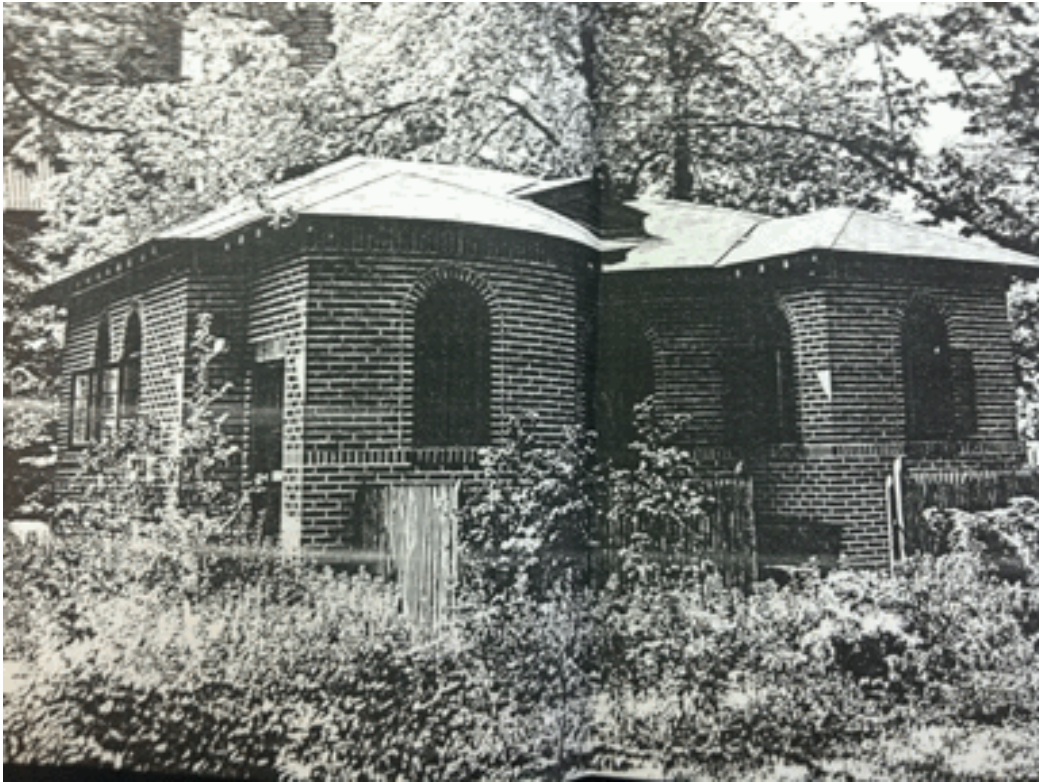
Figure 10. A new lodge house is constructed on Reservation 59 in 1930. This one-story brick building contained both men's and women's restrooms and space for the park police (National Mall and Memorial Parks Archives)
