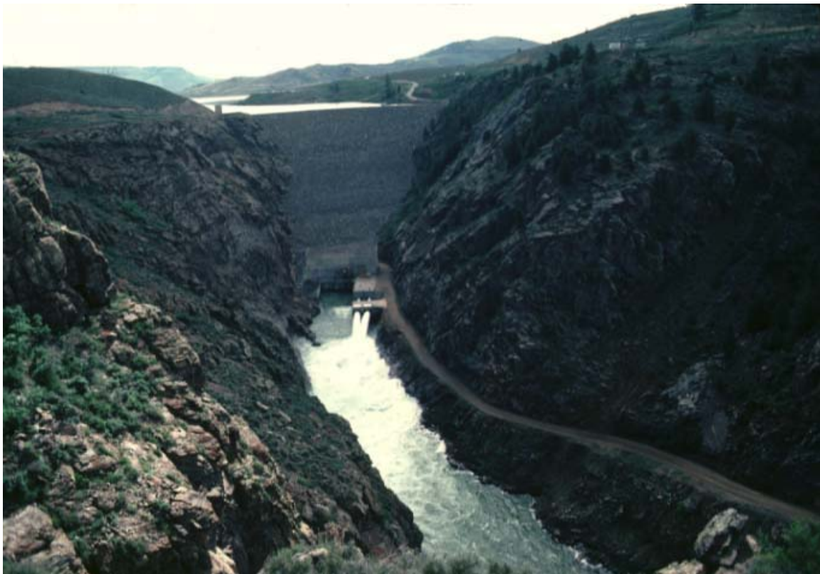
Figure 76. Blue Mesa dam releasing water through its jet tubes used during periods of large releases (photo: Reclamation).
