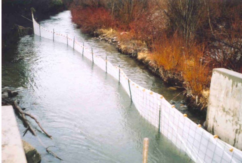
Figure 74. Screen set up by CDOW to divert stocked kokanee away from an irrigation ditch on the Gunnison River above BMR.
