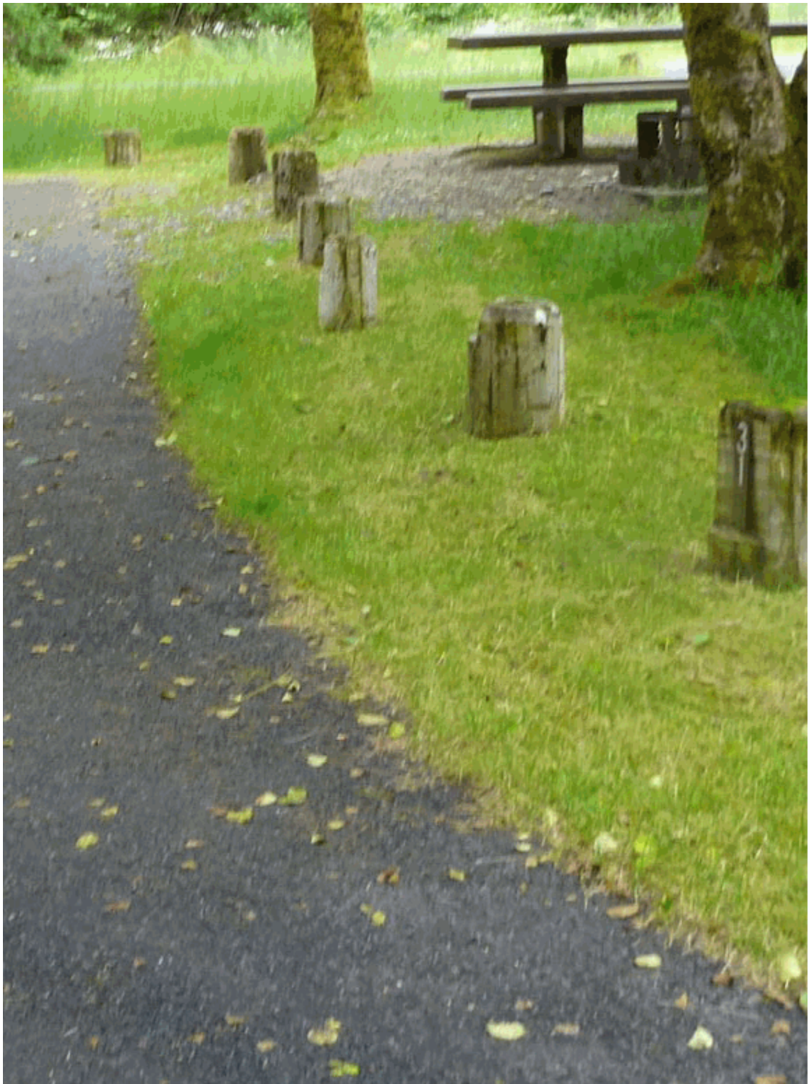
Photograph of the wooden bollards along a campground spur. These are a contributing feature of the original Mission 66 design. (PWRO 2012)
