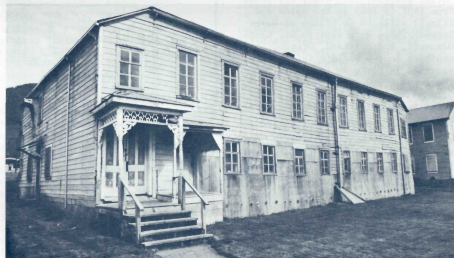
Top: Russian Bishop's House, 1885. Note the priest with the two children on the porch. Bottom: Pre-restoration Russian Bishop's House. Note the structural changes.
