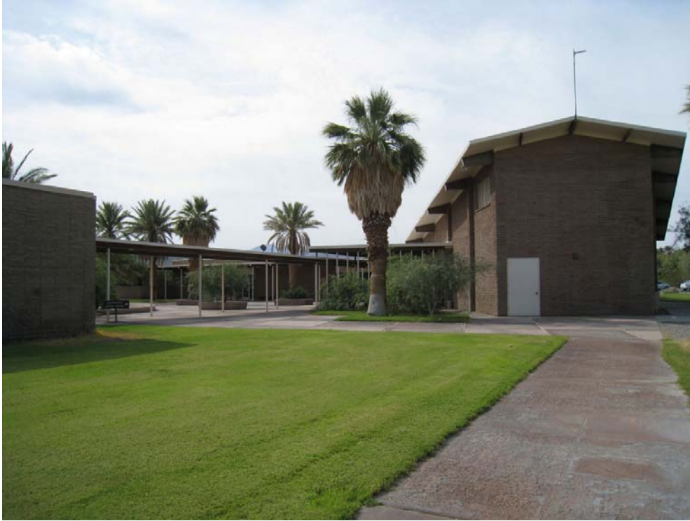
9. Auditorium, Furnace Creek Visitor Center Historic District, Erica Owens, June 2009, digital image (CA_InyoCounty_FurnaceCreekHD9_Auditorium.tif). North elevation of auditorium (left) and courtyard (right), looking south.
