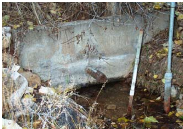
Figure 6. Sorenson spring was capped in the early 1900s and the water piped for agricultural and household use.
