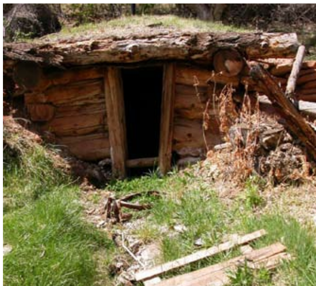
Figure 7. Lockhart ranch features a springhouse used to keep food cold.
