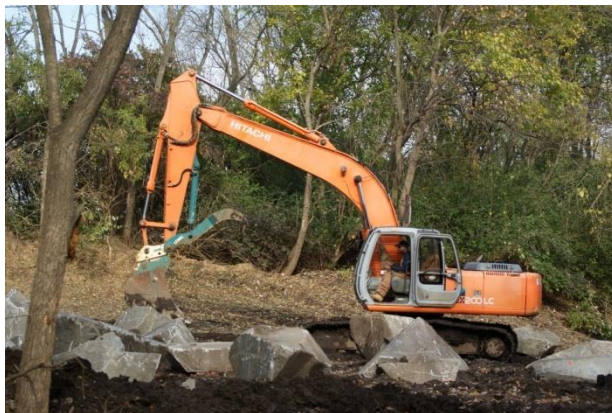
Construction of outdoor classrooms on Kingman Island
