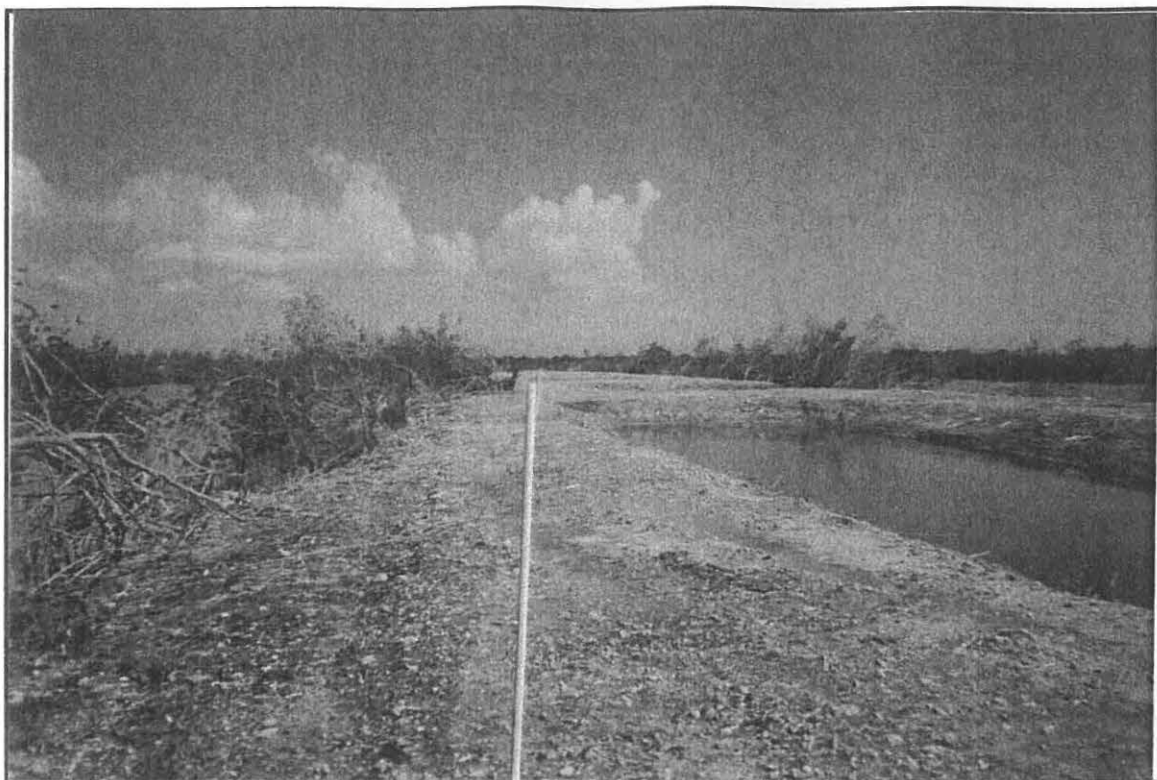
Date: March 1, 2006 Location: Cooling Canals Transect #3 Photo Station #3
