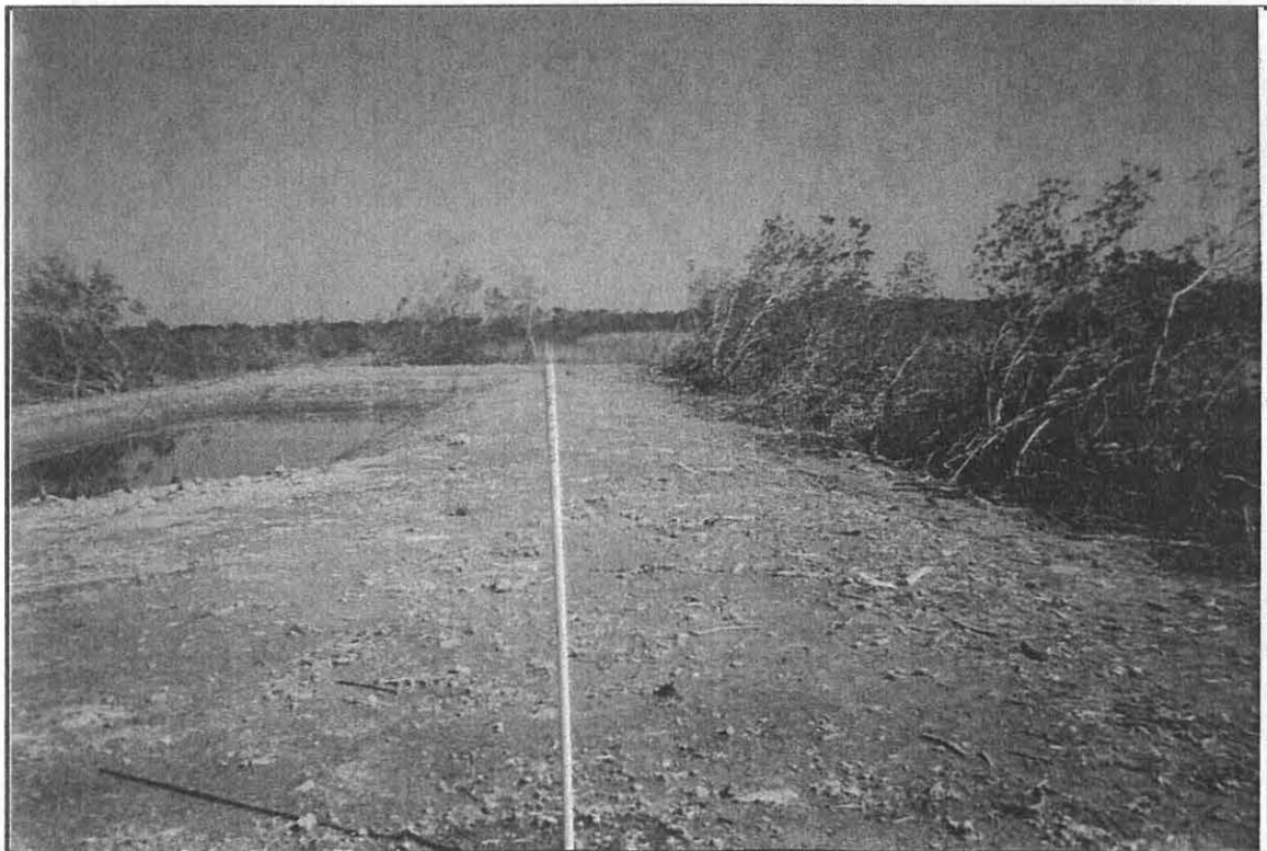
Date: March 1, 2006 Location: Cooling Canals Transect #10 Photo Station #10
