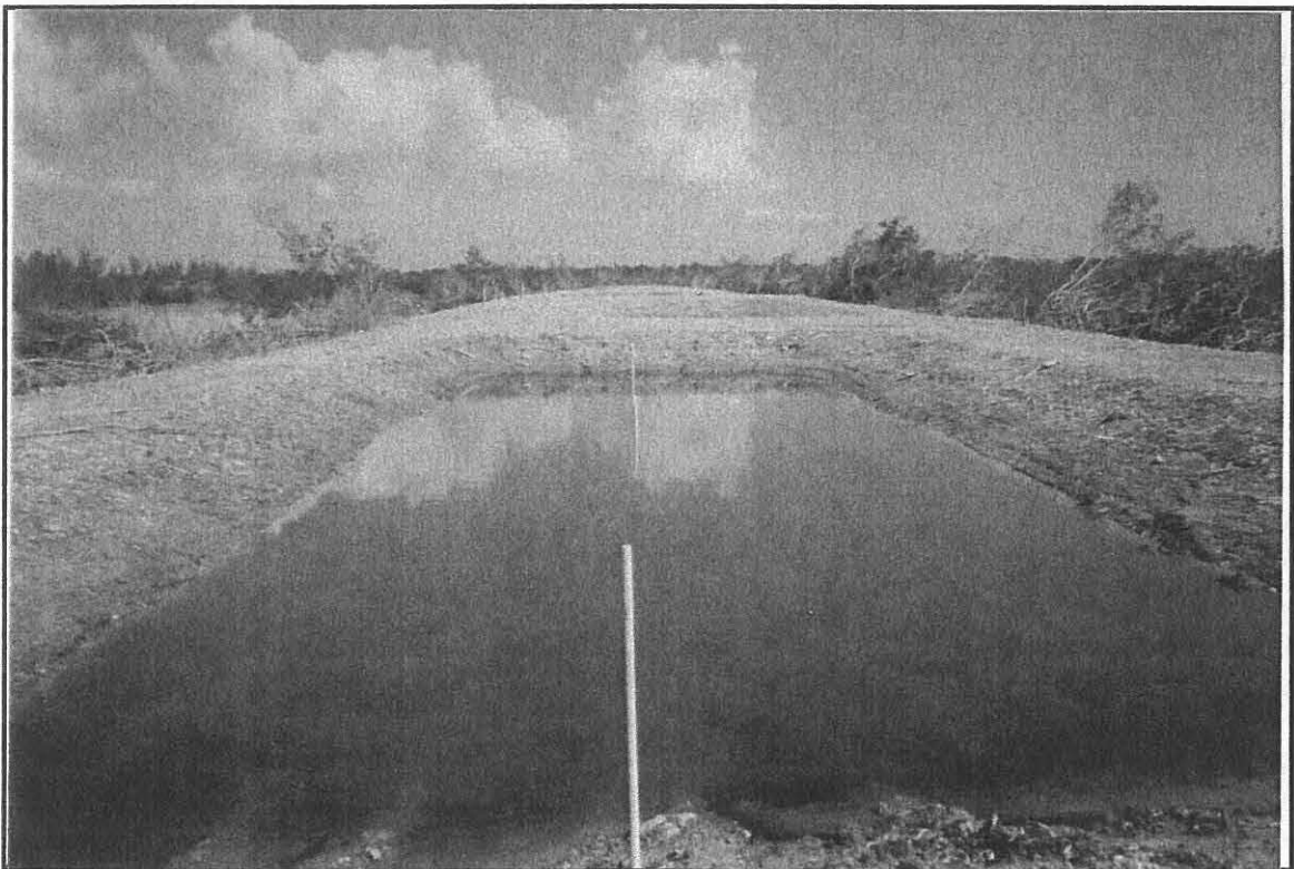
Date: March 1, 2006 Location: Cooling Canals Transect #4 Photo Station #4
