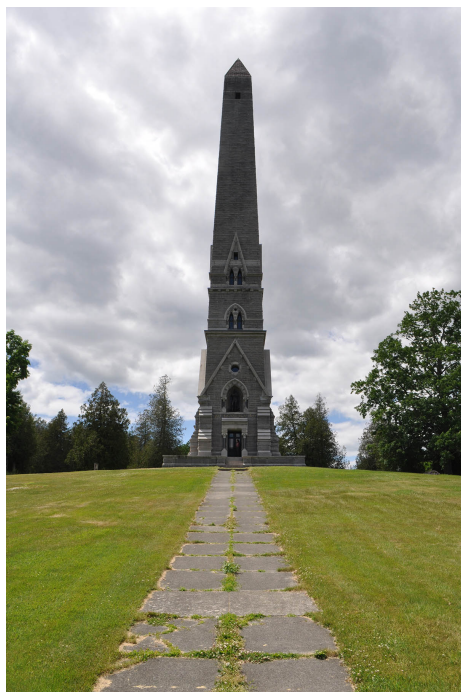
Figure 21. Saratoga Monument, view looking west from the east path. (OCLP 2022)
