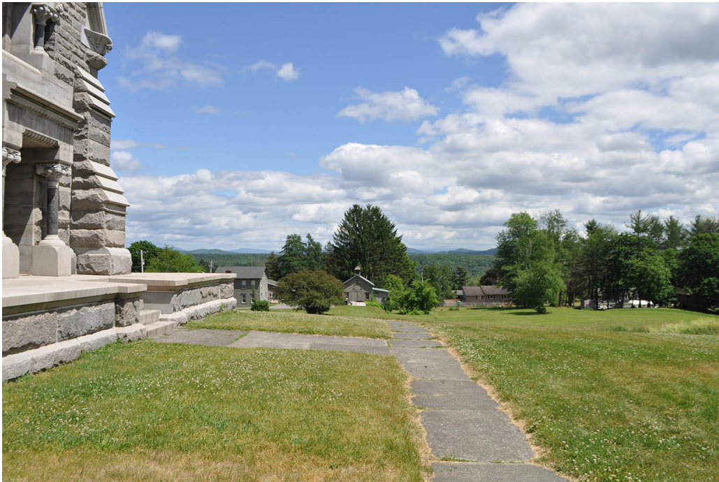
Figure 26. Historic concrete walks, view looking east from the southwest corner of the monument. (OCLP 2022)
