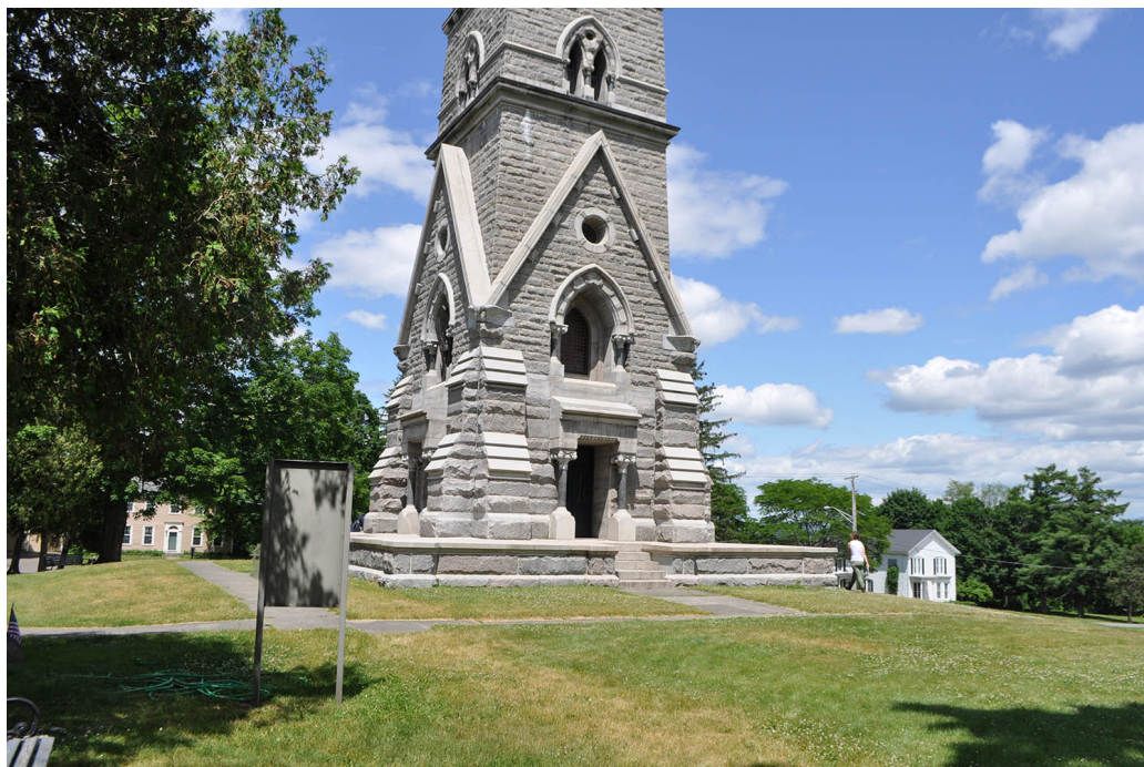
Figure 23. View looking northeast at walkways around the base of the monument. The worn grass area and asphalt path sit atop the former carriage road. (OCLP 2022)
