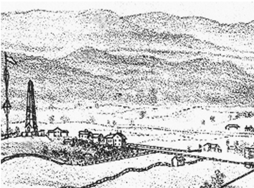
Figure 6. The Saratoga Monument under construction, 1877. Portion of birds-eye view of Schuylerville, NY drawn by Nathaniel Sylvester. Note the ship mast flagpole with the garrison flag. (Sylvester 1878)
