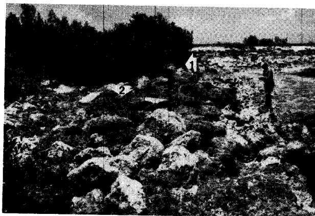
Ground view at McArthur Causeway, Government Cut, May 1980, showing a seawall and riprap. This is a heavily used boat channel. Oil penetration would be greatest in the coarse-grained gravel at the toe of beach (arrow 1). The dark band (arrow 2) is algae which was abundant and diverse in sheltered conditions where the substrate was stable.
