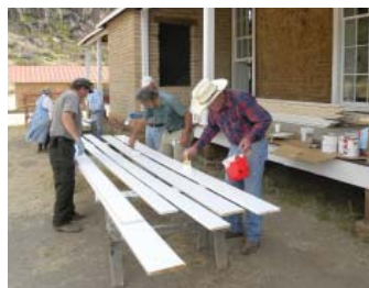
Painting of 2,400 feet of ceiling boards (2009).
