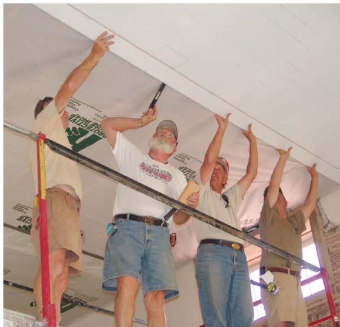
Installing the new ceiling in the north ward (2009).
