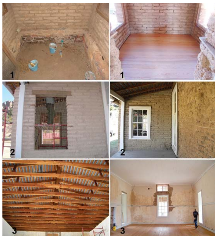
Before and after views of the north ward (1) addition of flooring in wash room (2) wash room window installation, and (3) new ceiling in the ward (2009).
