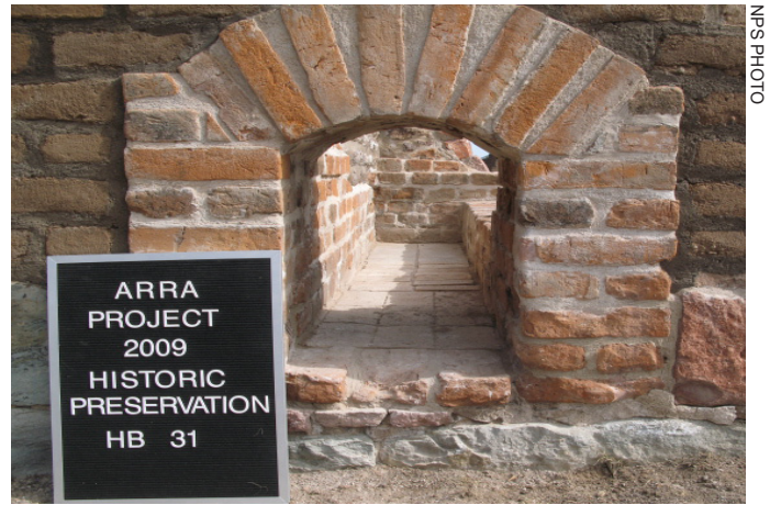
Part of a recently-restored oven at the post bakery.
