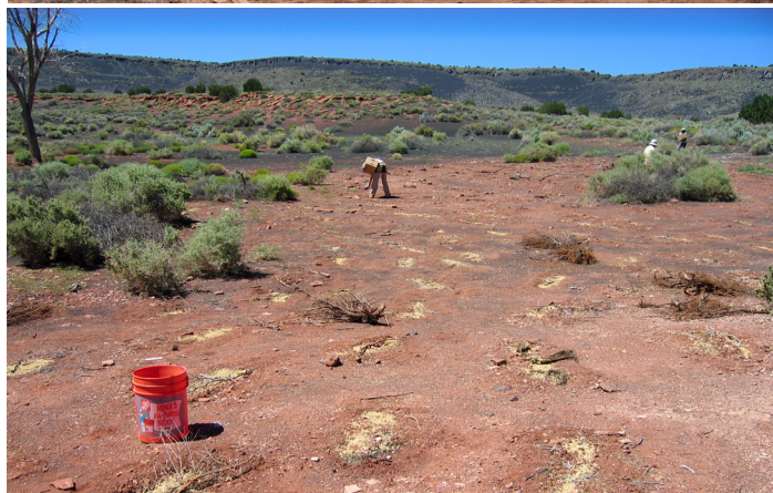
Pumpshack at Heiser Spring, before (top), during demolition and removal (center), and during revegetation efforts (bottom).
