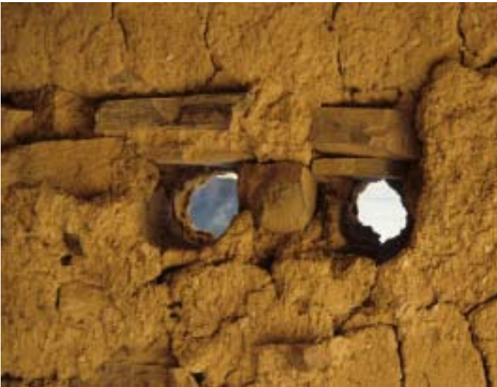
Wood in a wall at the Tonto Upper Cliff Dwelling.
