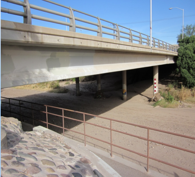
Congress Street Bridge on Santa Cruz River
