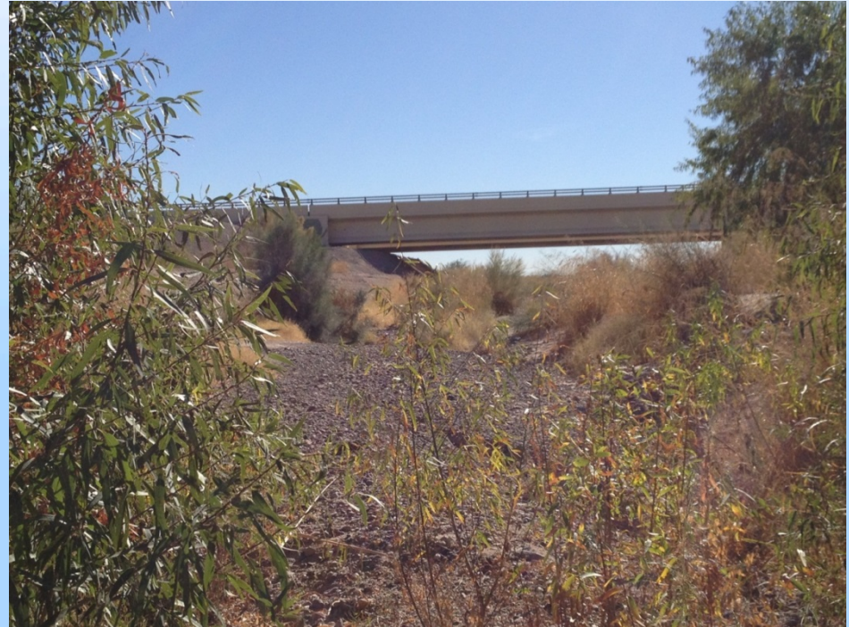
Twin Peak Bridge on Santa Cruz River
