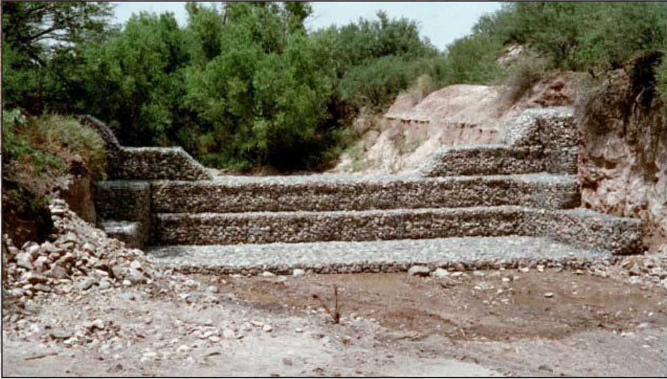
A San Bernardino gabion
