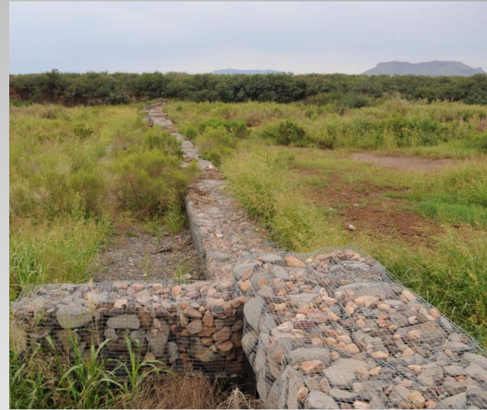
Rock basket gabions at San Bernardino Ranch, Sonora
