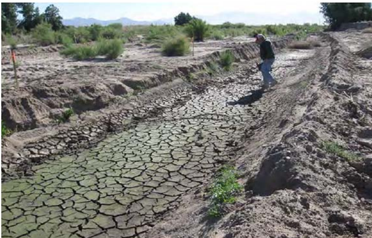
Photo 12. – Mudcracks in Channel 1 after 7 Days of Drying during First Maintenance Event. Brad Despaigne is crossing channel.
