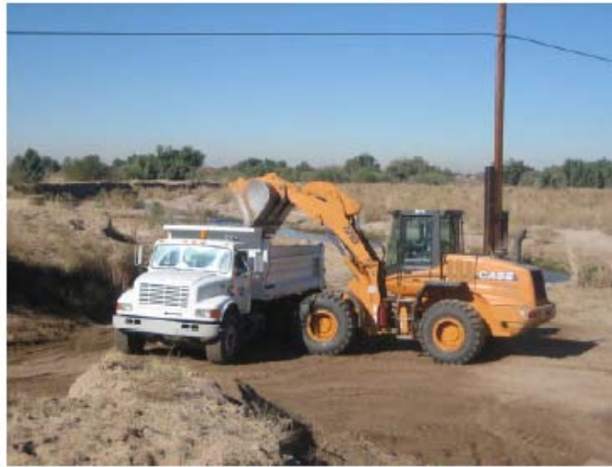
Photo 2. – Removal of Excavated Material during Excavation.
