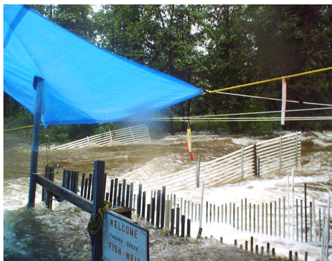
Figure 10. Tanada Creek weir at flood stage in 2005.
