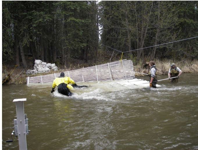
Figure 3. Constructing Tanada Creek weir, 2007.
