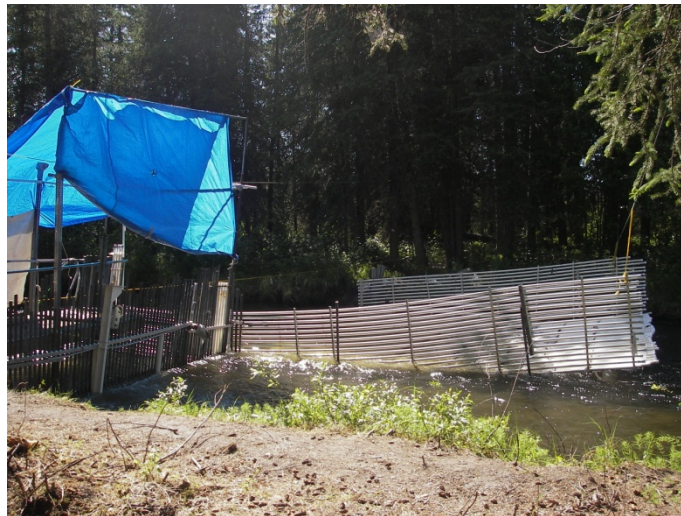
Figure 4. Completed Tanada Creek weir structure, 2007.
