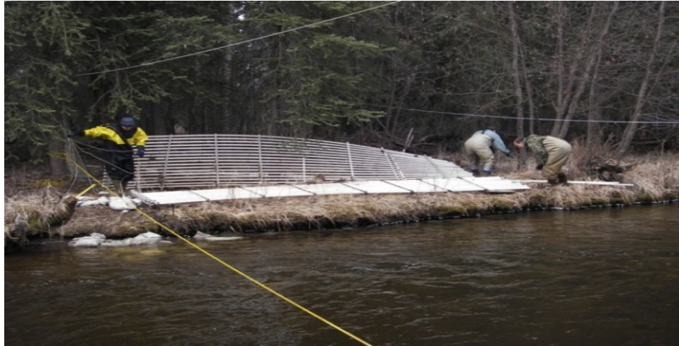
Figure 3. Constructing Tanada Creek weir, 2008.
