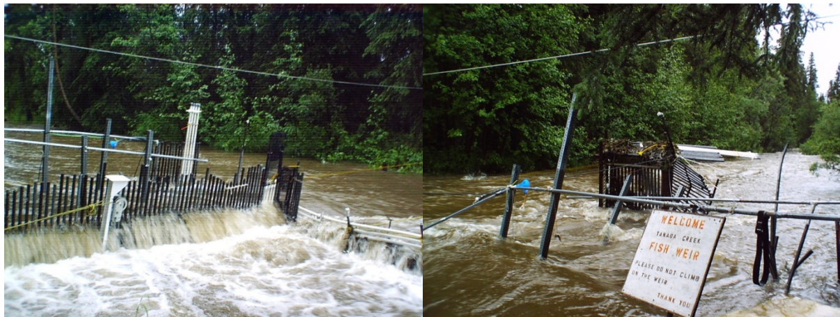
Figure 10. Tanada Creek weir at flood stage, July 8-9, 2008.
