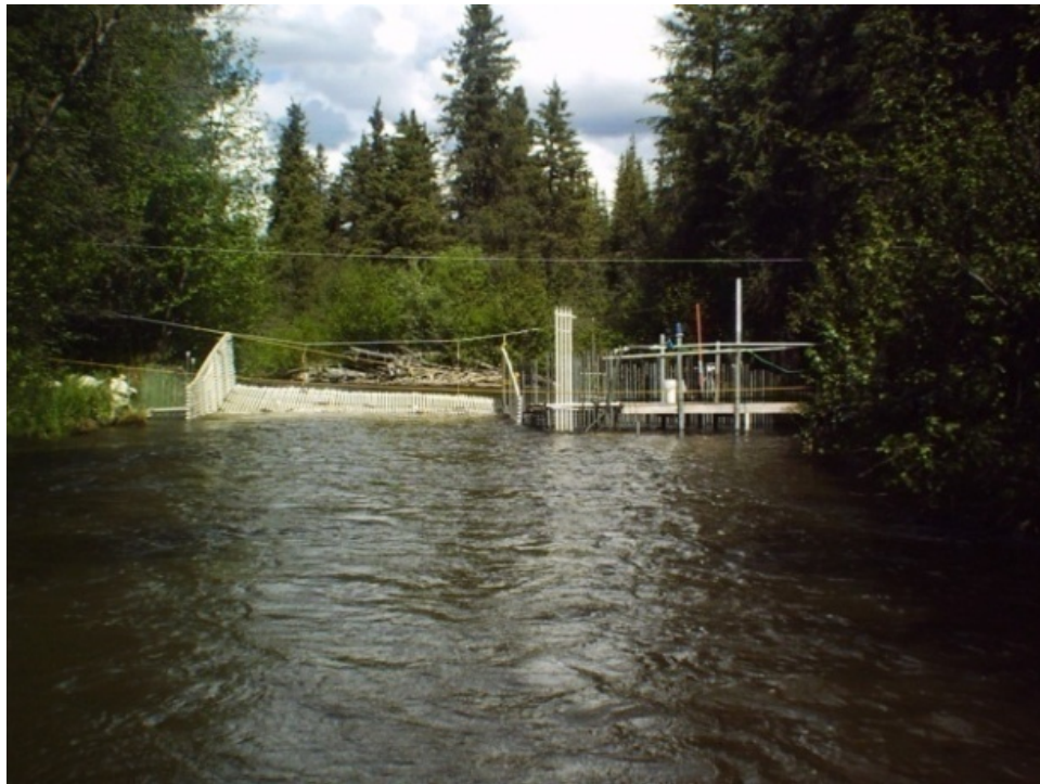
Figure 4. Completed Tanada Creek weir structure, 2008.
