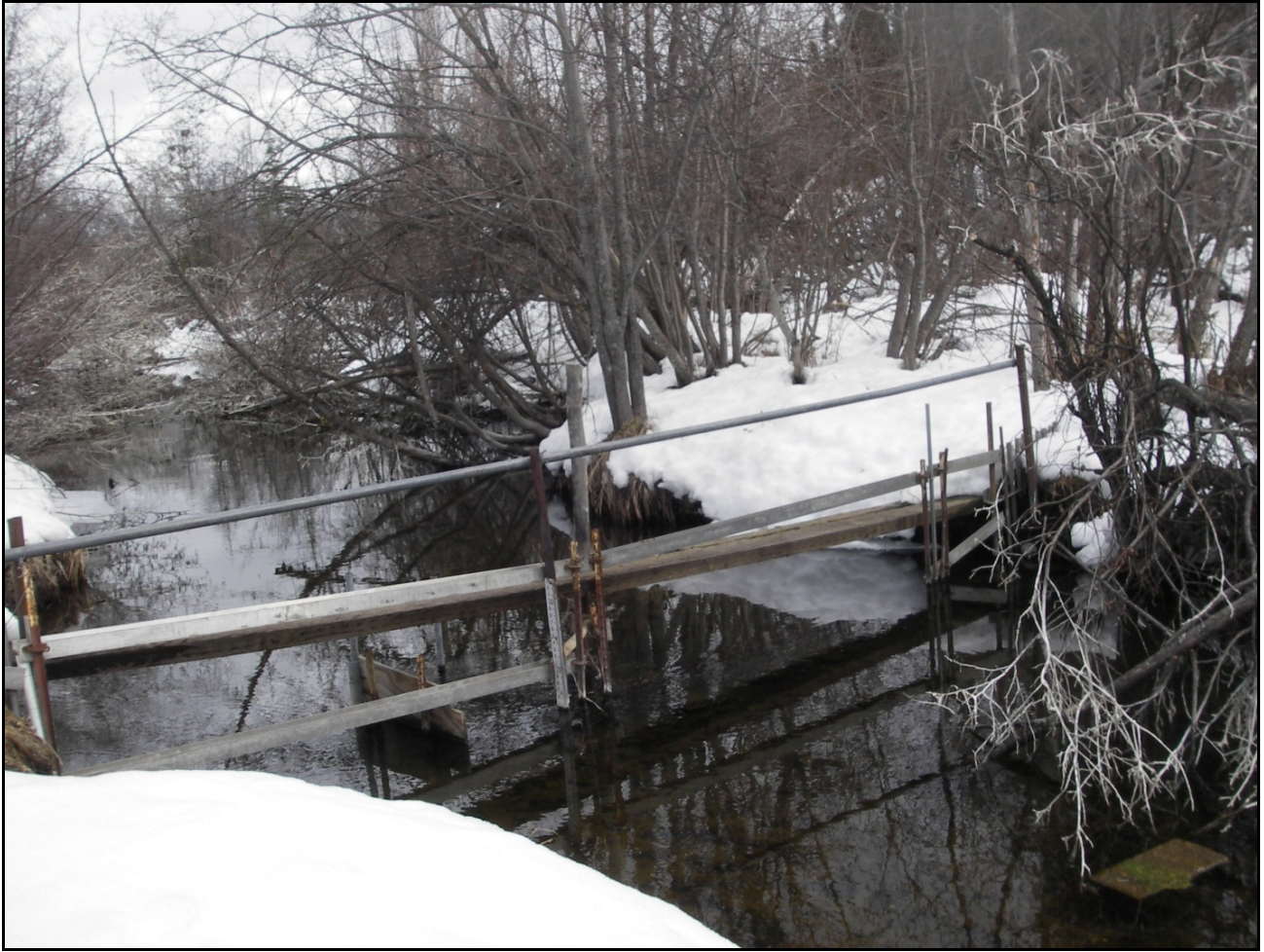
Figure 17. Long Lake weir, April 2006.
