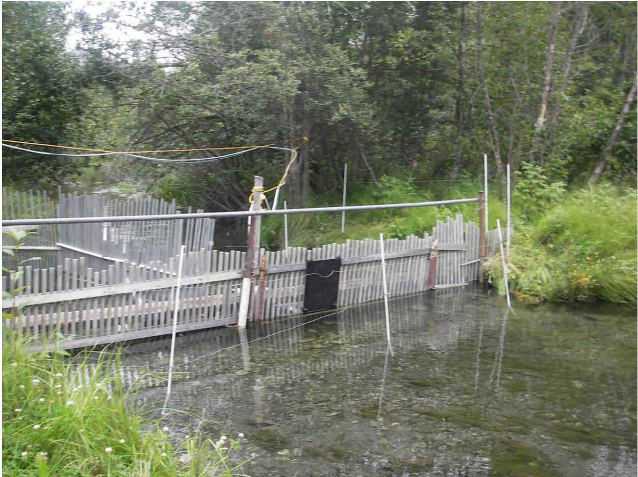
Figure 3. Long Lake weir with video installed.
