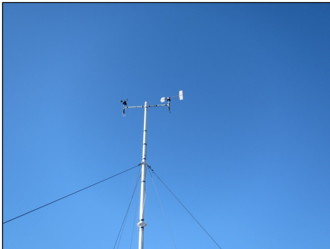
Figure 30. Harding Icefield RAWS – Wind direction sensors after unscheduled repairs.
