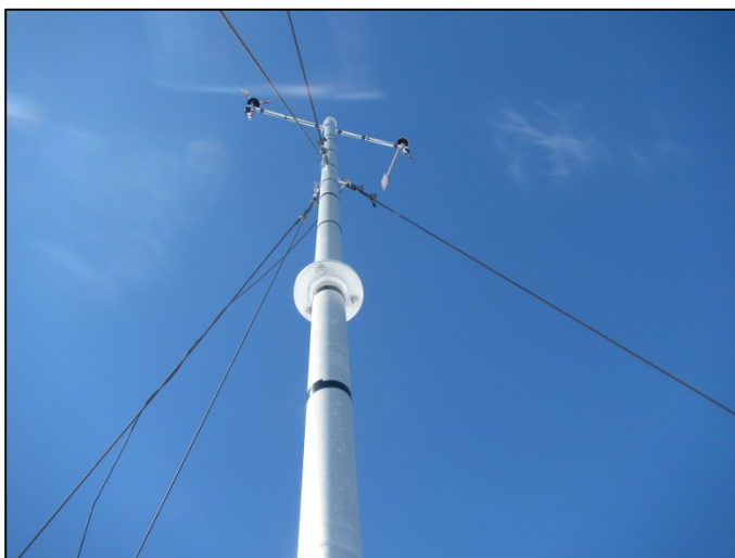
Figure 24. Harding Icefield RAWS – Wind direction sensor without tip and broken guy-wire.
