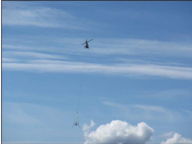
Figure 31. Hickerson Lake RAWs – Helicopter sling load of Hickerson Lake weather station frame.
