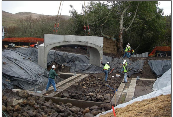
Workers place a piece of the bottomless culvert at the Estero Road crossing.
