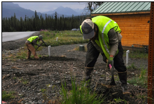
Figure 15. SCA Crew members use pulaskis to reduce the amount of soil compaction in the revegetation area near C-Camp
