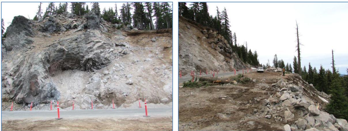
Figure 1. Disturbance to road shoulders and road cuts from the 2014 Rockfall Mitigation project. Photos by Kathryn Williams.
