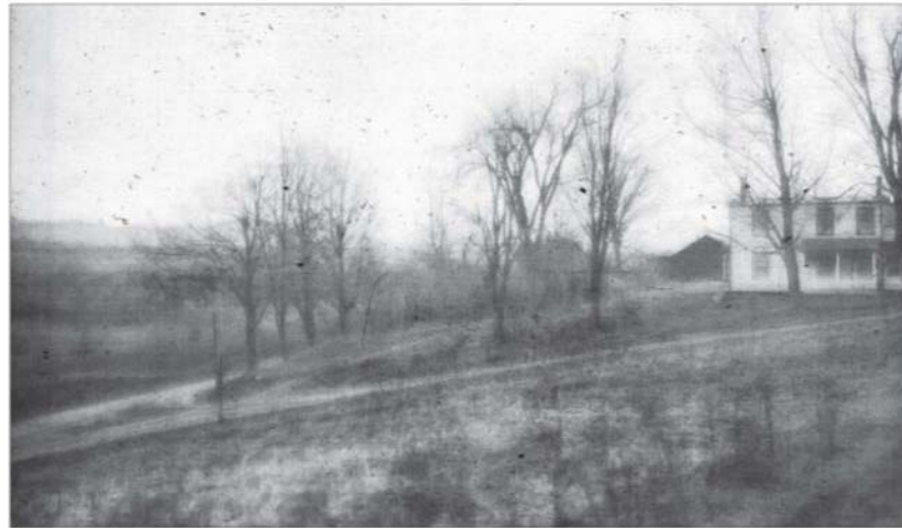
Figure 1.25. Enhanced negative. View of George Hathaway house (Germain house) property c. 1920s. To the left is the intersection of Chubbs Hill Road (Schuyler Street) and the Whitehall Turnpike (US Route 4). Open fields in front of the house depict it as agriculture. There is no sign of trolley tracks and the size of the negative suggest pre-1900 (SARA).
