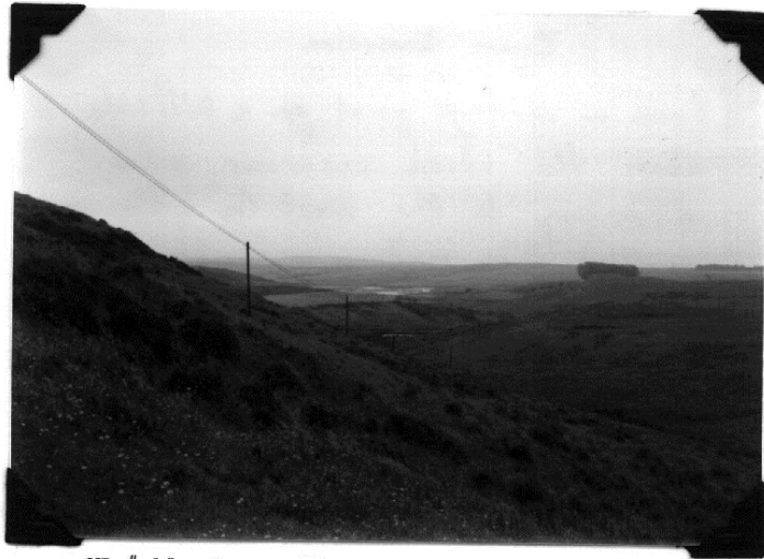
WR # 10 - Rogers Diversion From a vantage point on a hillside above the stock reservoir, view is looking to the West (a little south.) The roadway is visible in the center and the western portion of Point Reyes in the background. July 8, 1975
