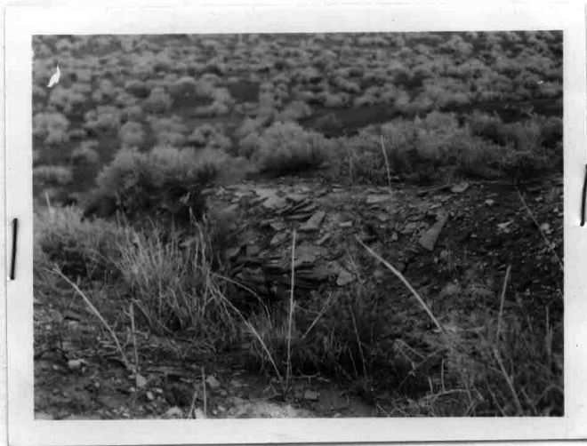
WUP-47-D-1 - Trench at Wupatki Spring Diversion
