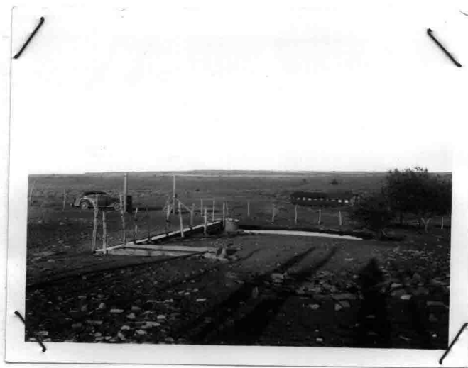
WUP-47-D-3 - Pond and CCC Barracks at Heiser Spring - Heiser Wash drains to left of Barracks - July 1947
