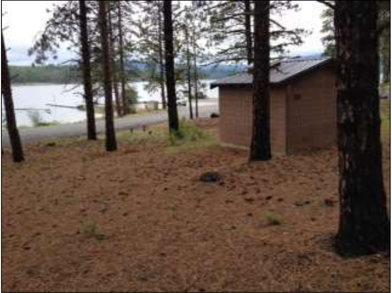
Figure 2. The water-supply well at Gifford campground is located inside the cinder block building. The boat launch ramp and dock are in the background.
