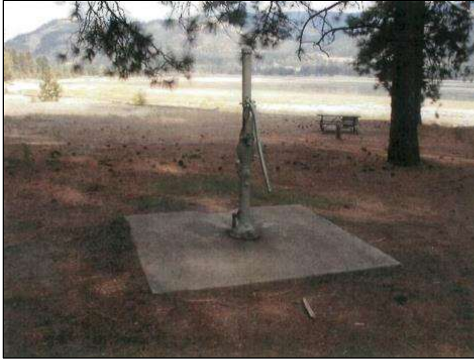
Figure 2. Hand pump on well at Haag Cove campground.
