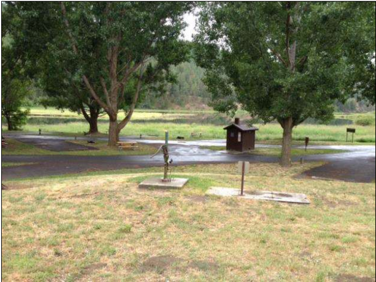
Figure 2. Hand-pumped well at Hawk Creek campground. Iodine treatment chamber is in a cinder block vault to the right of the well. Normal full-pool shoreline is on the far side of the paved road, 145 feet from the well.
