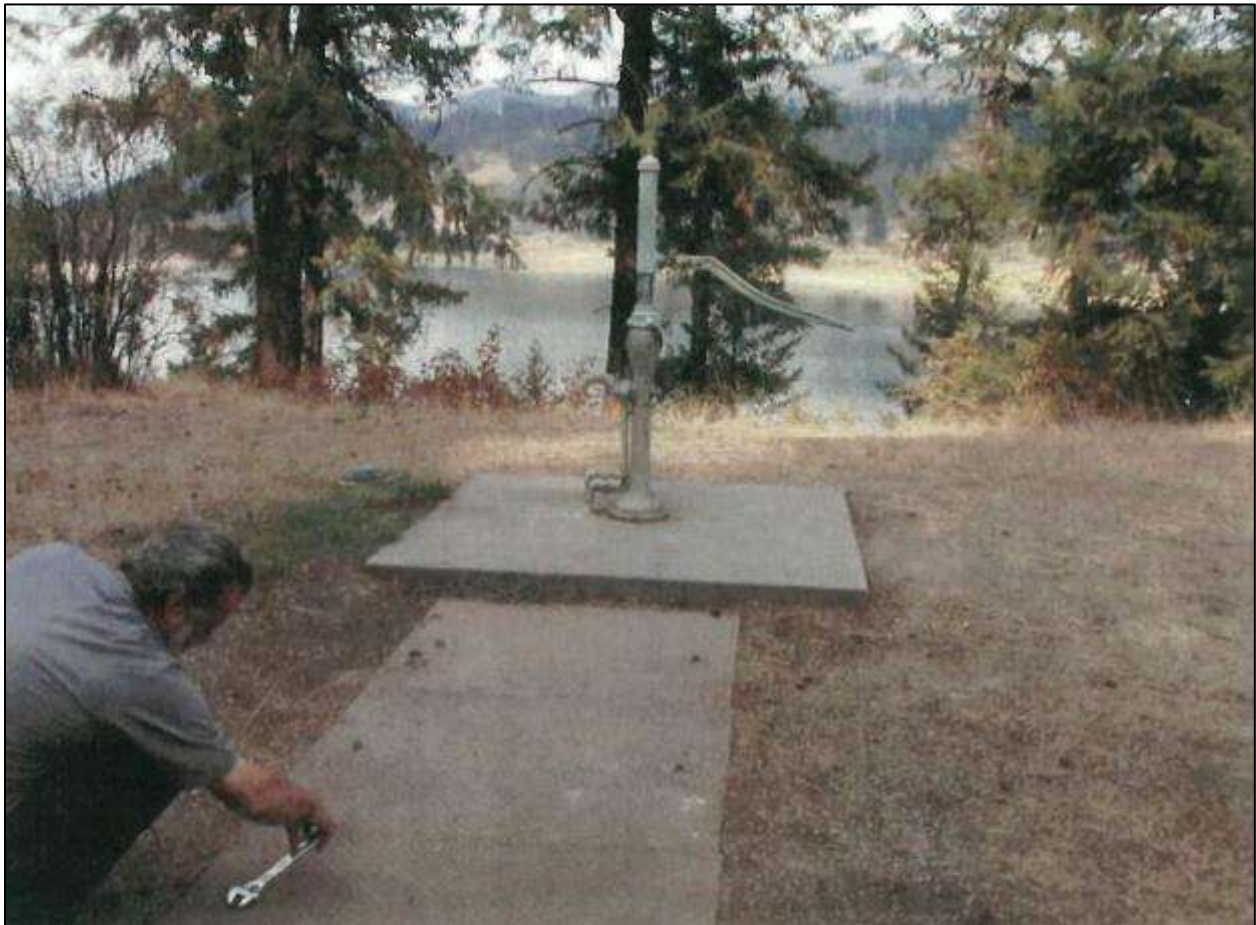
Figure 2. Hand pump on well at Kamloops campground. The iodine treatment and contact chamber are in the vault in the foreground of the photo.
