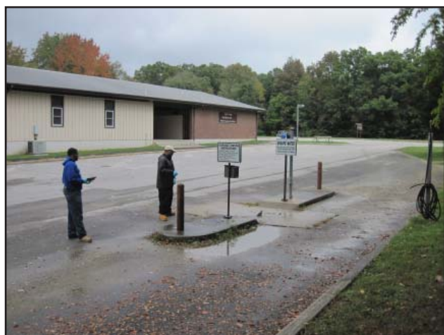
Figure 1: Storm-water drains from the Post Office parking lot and mixes with spilled waste residue, rich in QAC, at the RV disposal station. It carries the QAC into the storm filter, down the ravine, and into Annette's Dome (Cave level B). This drain area needs to be re-designed to prevent chemicals from getting into the cave.
