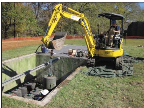
Figure 1: Contractors serviced the storm-water filters by swapping the cartridges. (Hotel-east shown here)
