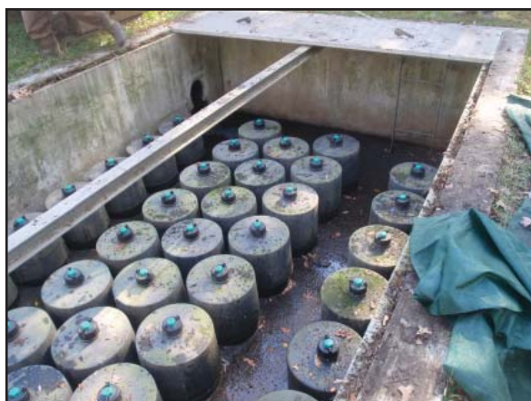
Figure 1: ZPG cartridges in filter system.
