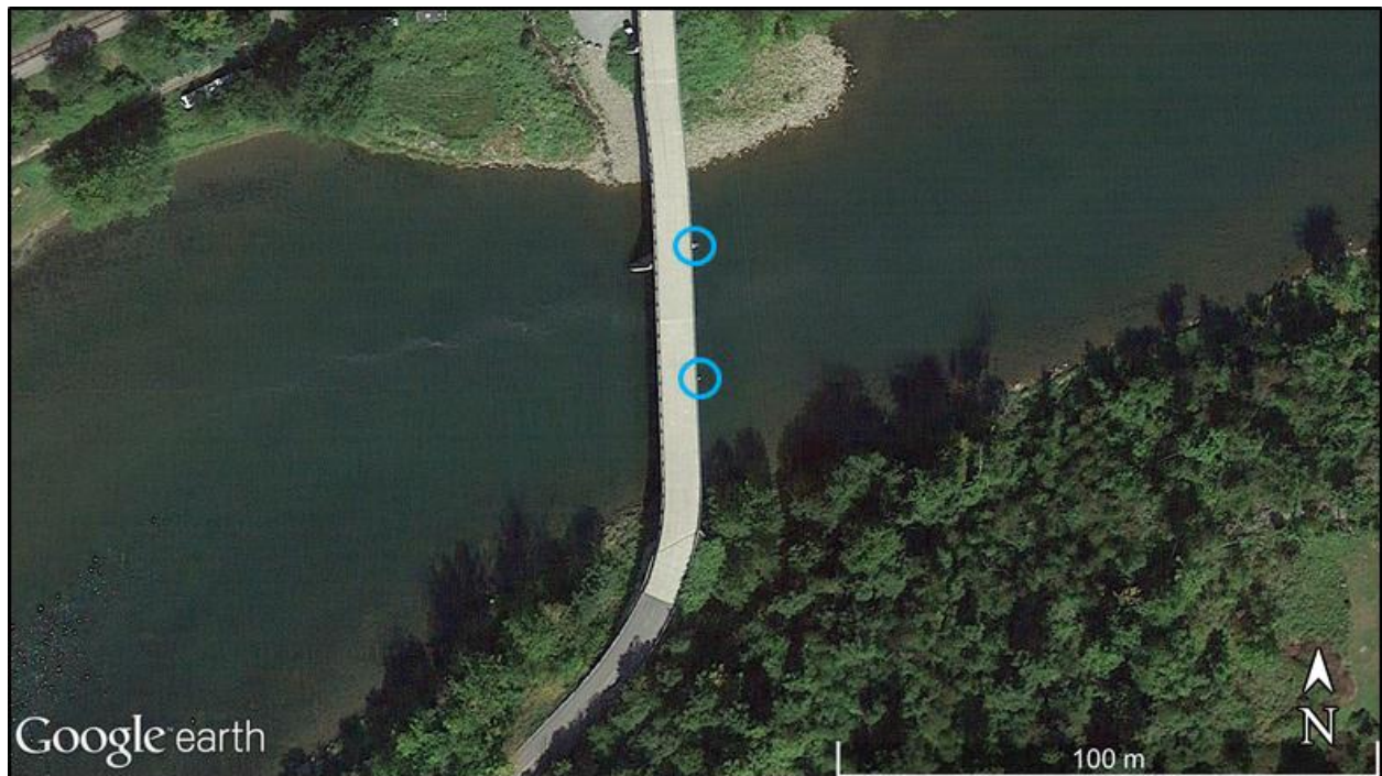
Figure 2. Aerial view of Lordville Road Bridge across Delaware River near Lordville, NY. The top circle, located near the primary river flow, outlines the Eastern Rivers and Mountains Network water quality monitoring equipment whereas the bottom circle outlines the United States Geological Survey river stage recorder.
