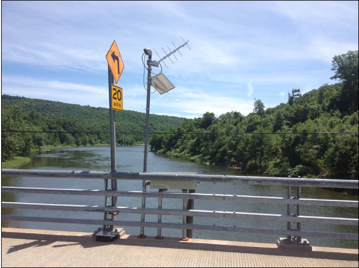
Figure 3. Photograph of Delaware River water quality monitoring equipment on the Lordville Road Bridge near Lordville, NY. A data collection platform that controls the datasonde is located within the aluminum shelter. All electronics are powered by a solar-charged battery and data are transmitted hourly via satellite and the pictured antenna.
