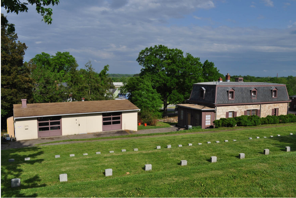
Figure 19. View looking east towards the lodge grounds and service yard. Shown in the image is the garage/equipment shed (c.1960) and the lodge (c.1870) (OCLP, 2011).
