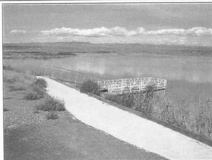
Photograph 3. Dog Creek Reservoir showing accessible fishing pier and footpath.
