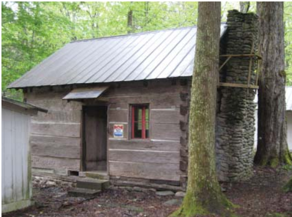
Figure 3, Southwest oblique view of the cabin.
