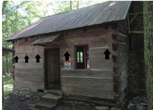
Figure 4, Notches on west elevation suggest a previous porch.
