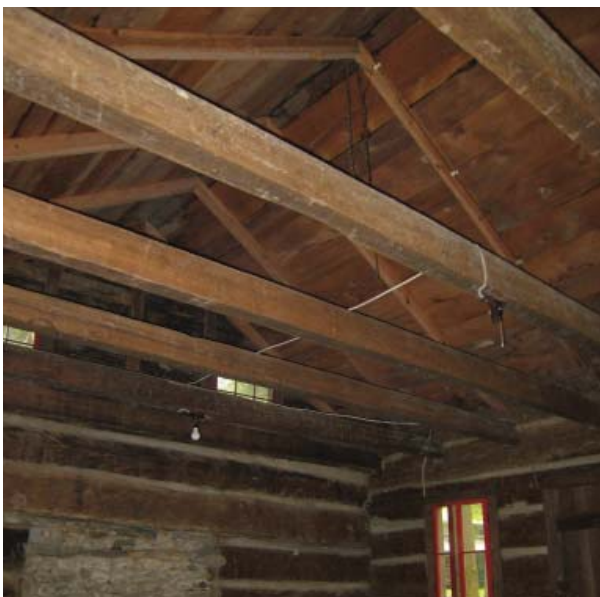
Figure 10, View of exposed roof structure.
