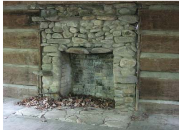
Figure 27, River stone fireplace with brick firebox constructed on the south elevation in 1932.
