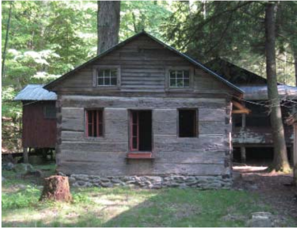
Figure 23, All five windows of the north elevation were reportedly added during the 1932 reconstruction. Only one window opening, probably on the west elevation, is original.
