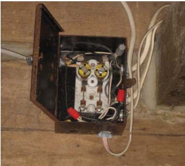
Figure 13 , Early fuse box on the interior surface of the west wall of Trentham Cabin.
