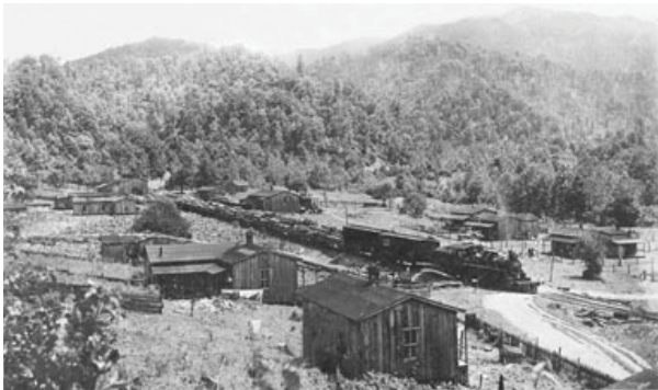
Figure 10. Undated photograph of log train in Elkmont. (Little River Lumber & Railroad Museum)
