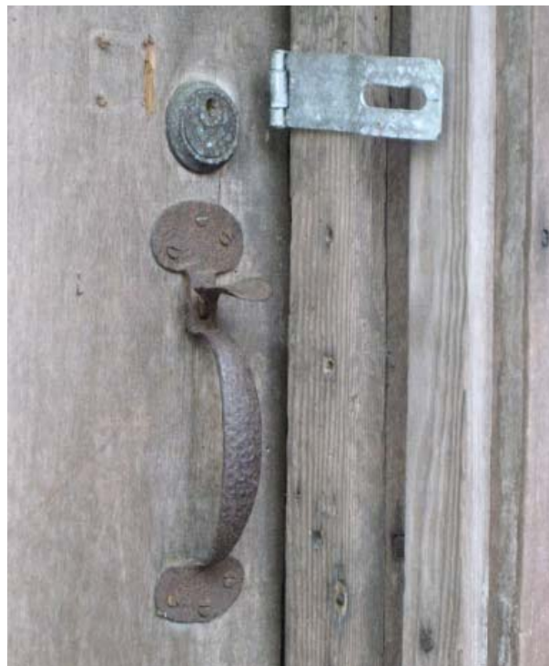
Figure 18, Wrought handle at west elevation front door.
