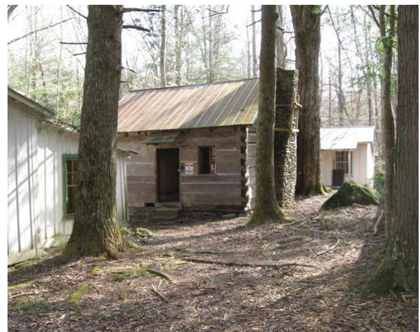
Figure 2, View of Trentham Cabin between Mayo Cabin in foreground and Servants' Quarters behind (photo from Diane Flaugh, Cultural Resources Department, NPS).
