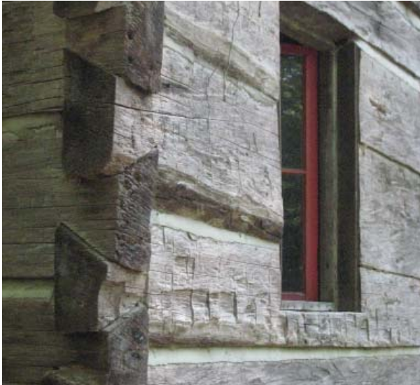
Figure 9, Half-dovetail notching at log corners.
