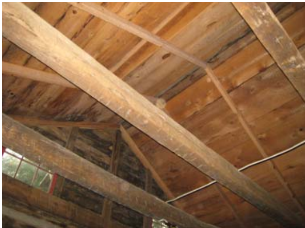
Figure 26, Exposed collar ties and roof rafters.
