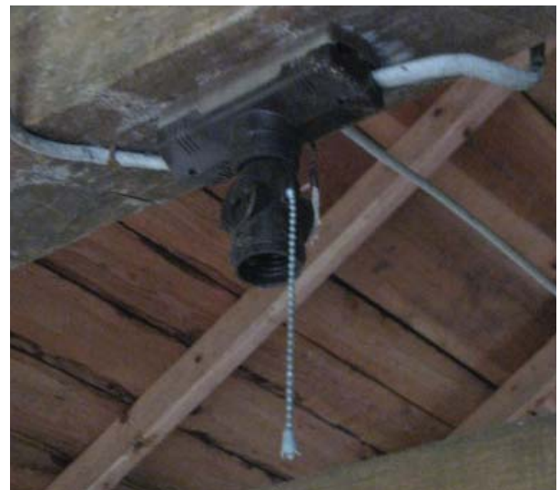
Figure 15 , Early Bakelite Corporation ceiling-mounted light fixture inside of cabin on bottom of collar beam.
