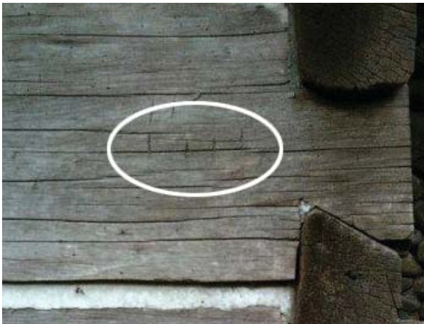
Figure 6, Identifying Roman numerals cut into the Trentham Cabin logs.
