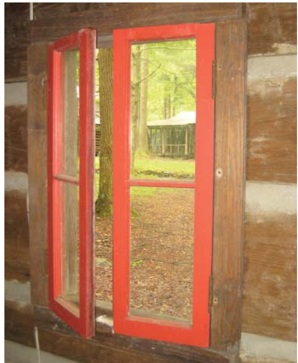
Figure 22, Typical paired casement window. Casing constructed in 1932 from floor boards from the Bogalusa Sawmill.
