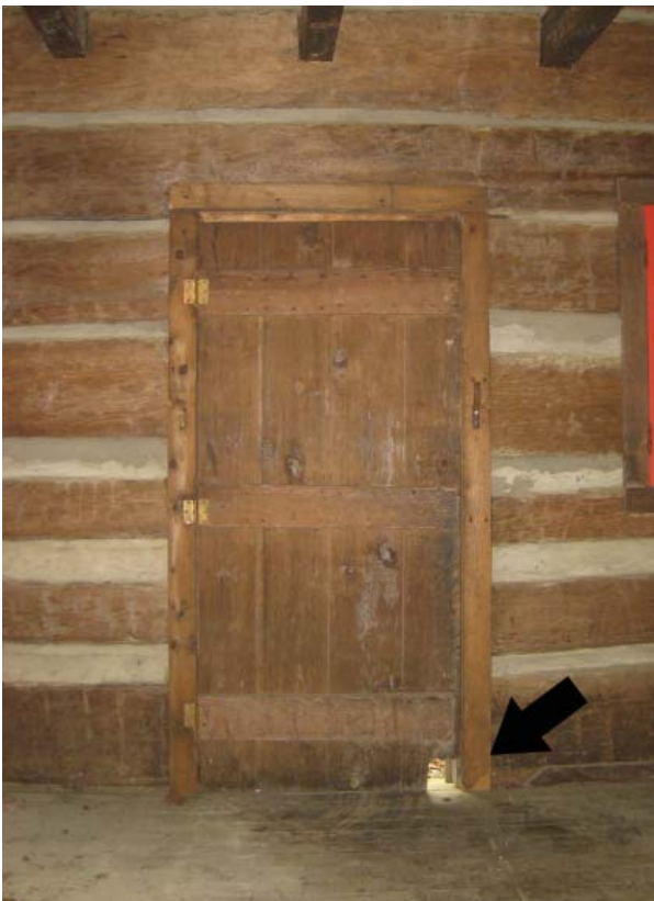
Figure 20, Interior side of east entrance door with corner notch for passage by the cat. Door is a 1932 reconstruction.
