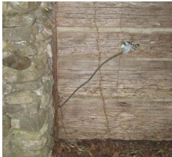
Figure 11, Gas line connection at south wall.
