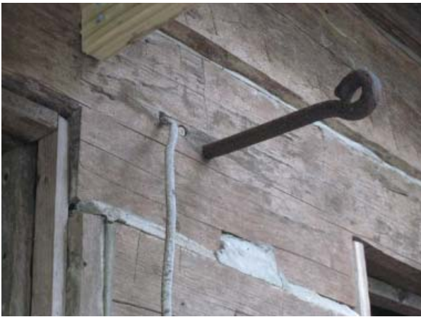
Figure 19, Hammered metal rod probably held an exterior lantern.
