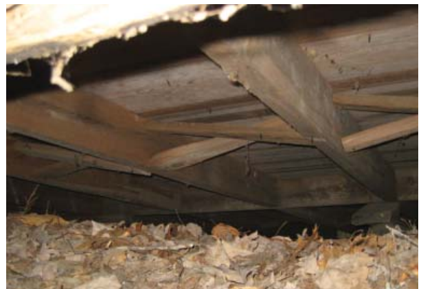
Figure 8, Modern conventional floor framing and flooring, both with Bogalusa Sawmill stamp, installed during 1932 reconstruction.
