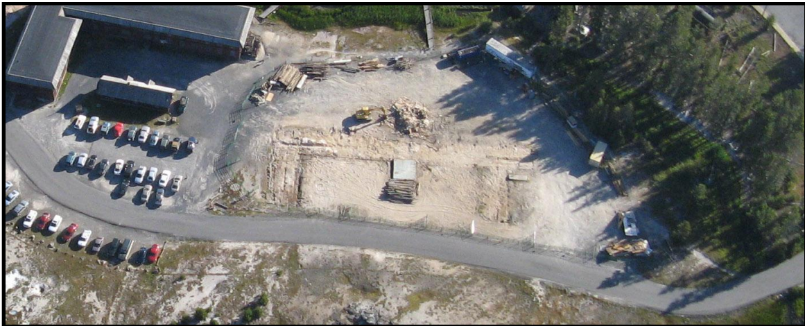
Figure 2. Aerial view of the historic Old Faithful pub taken on 20 August 2009. The complete removal of the building as part of the historic renovation allowed a detailed ground temperature survey. The outline of the former building can be seen in the center of the photograph. View is to the northeast.
