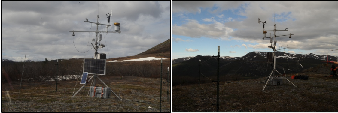
Figure 11. Salmon River, June 5, 2015 before (left) and after (right) repairs.
