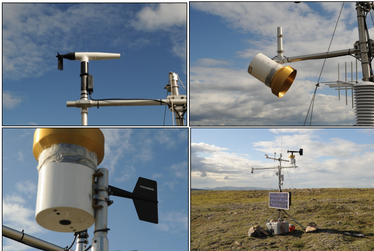
Figure 8. Kaluich, July 21, 2015. Clockwise from top: damaged WS-WD sensor, damaged RG-TB mount, repaired RG-TB mount, site after maintenance and repairs.
