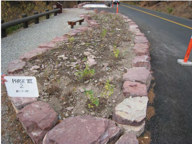
Planting Area 2 (St. Mary Falls TO west) photo 1 – 2015
