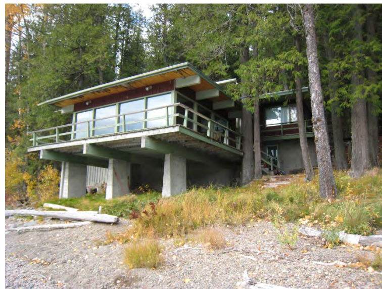
Photo 6. Moberly Cabin; wetland line is through pilings of foundation.
