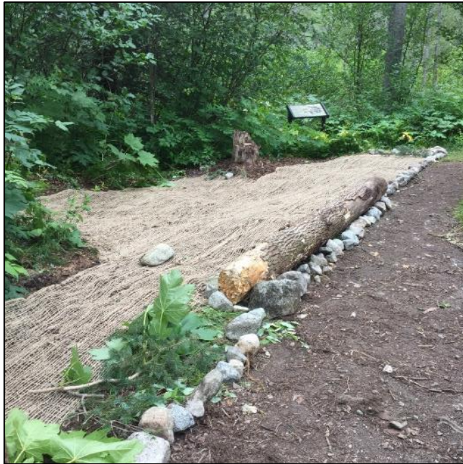
Figure 22. A large area of restoration across from warming shelters and southeast of the bear boxes.
