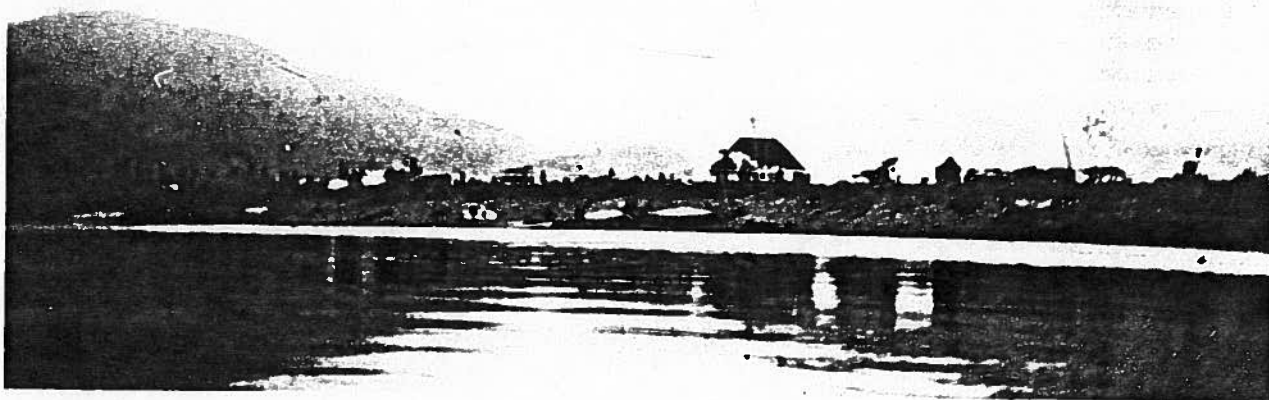
View of Shungnak from the Kobuk River, river in foreground. Kobuk District, Northern Alaska Region, Alaska. 1910. P. S. Smith. Courtesy USGS Historical Photo Library, Denver, Colorado.
