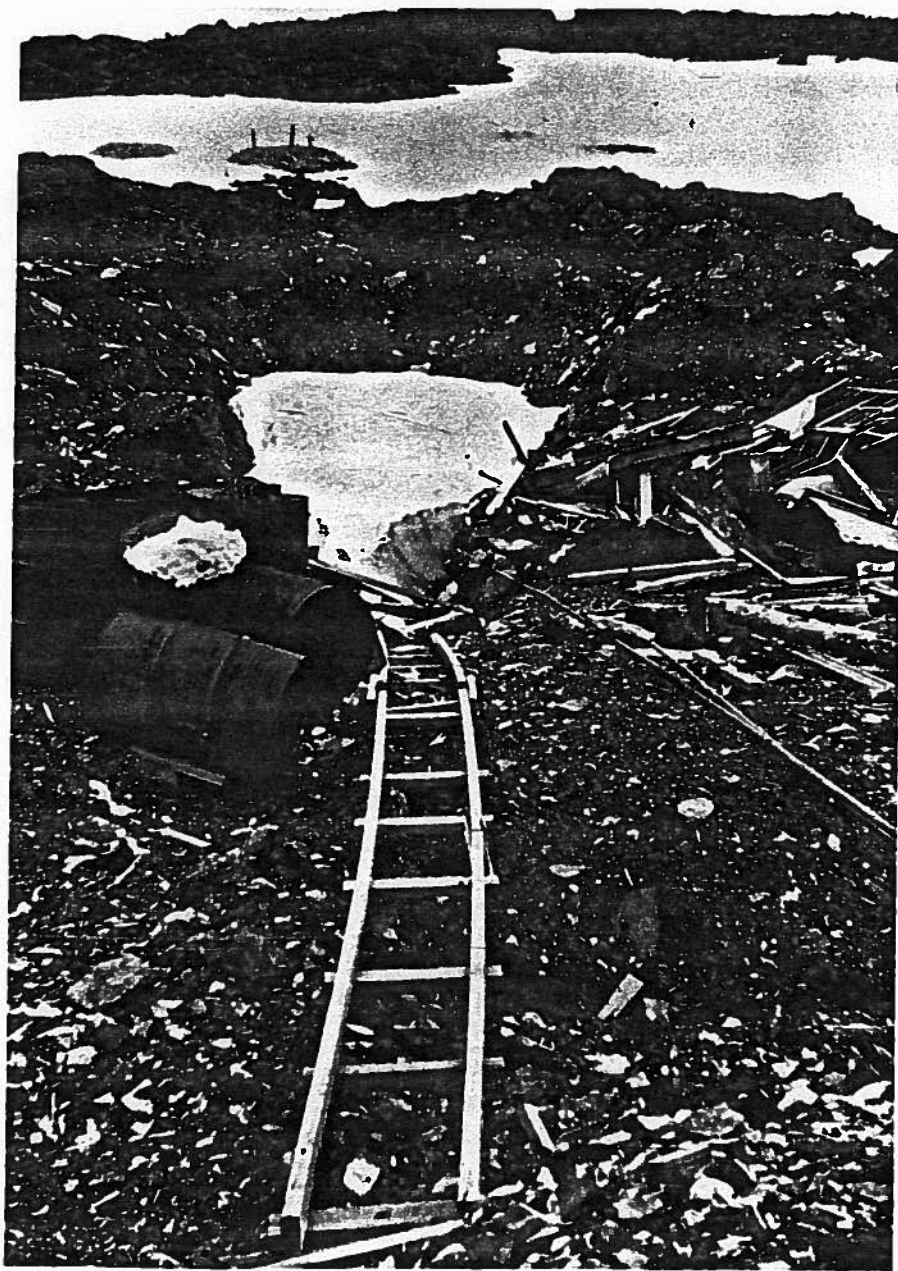
Entrance to Ingnik asbestos mine. 6/29/55. Irv Tailleir. USGS, Alaska Geology Branch.
