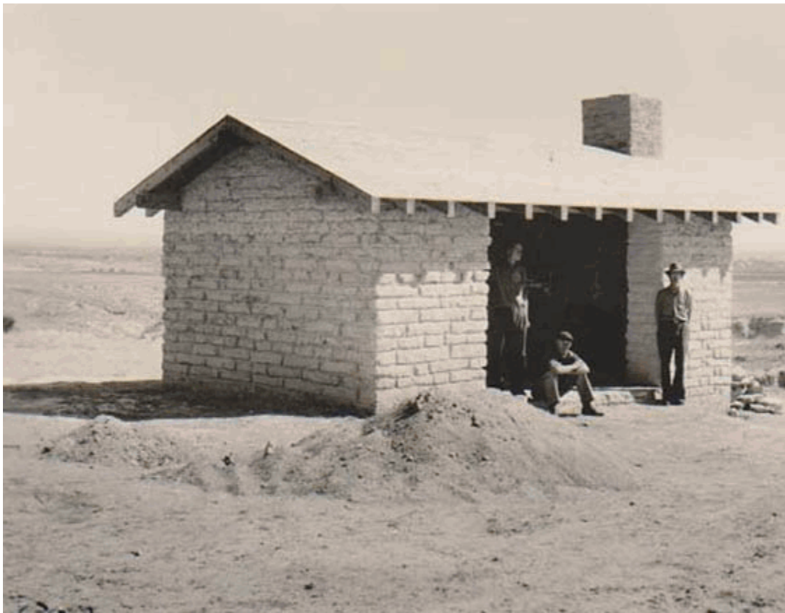
Gering Golf Course Shelter House in 1937. Image courtesy of Scotts Bluff National Monument.
