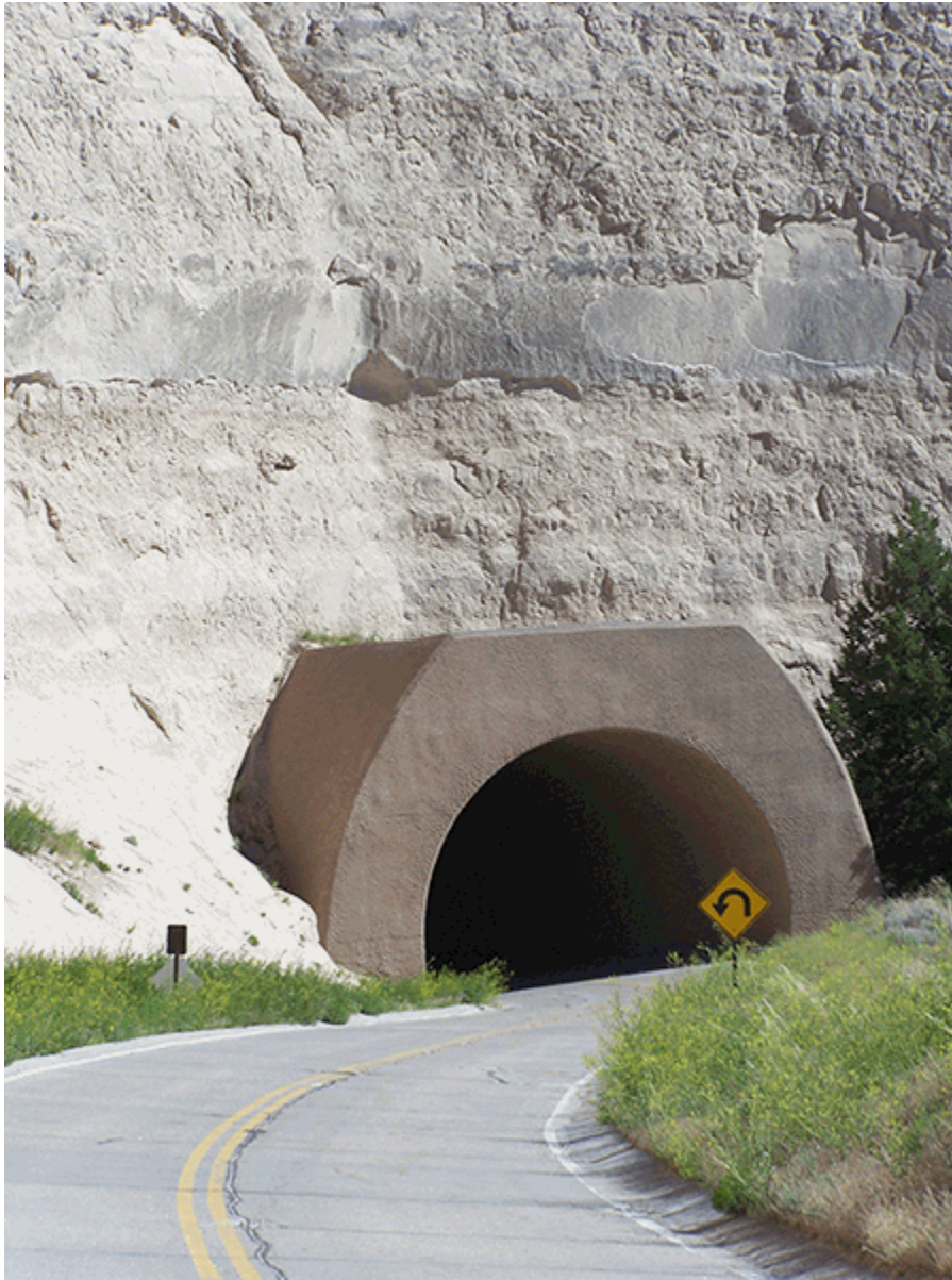
Summit Road Tunnel 1 looking south (Reed 2014).
