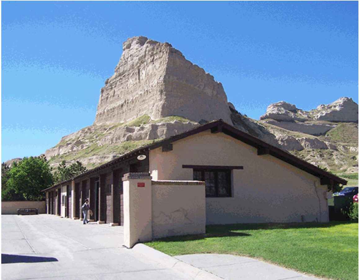
Utility/Maintenance Building looking west (Reed 2014).
