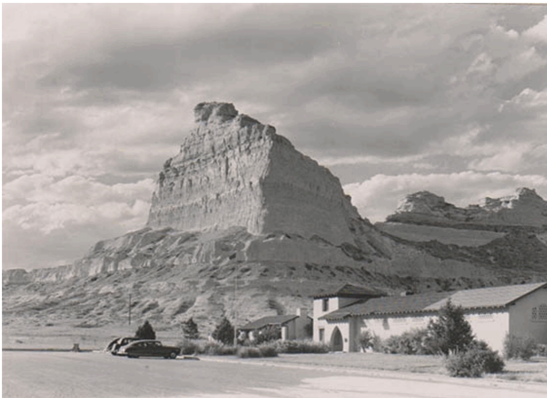
Scotts Bluff National Monument Visitors Center complex on August 24, 1949. Image courtesy of Scotts Bluff National Monument.
