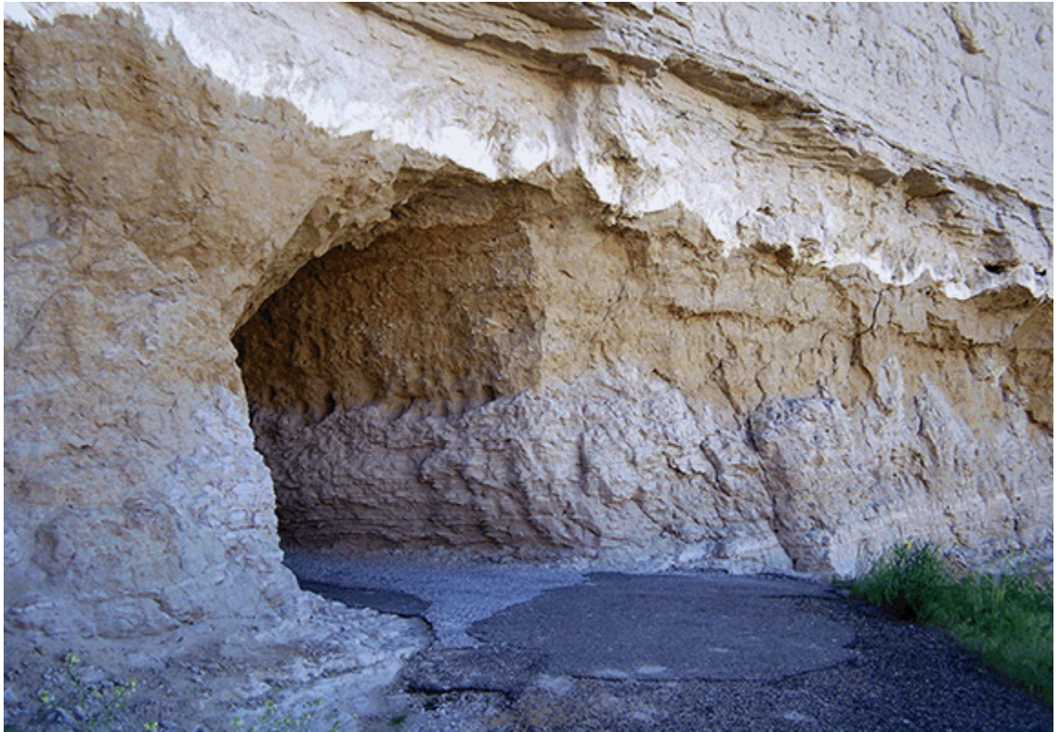
Saddle Rock Trail Pedestrian Tunnel looking northeast (Reed 2014).
