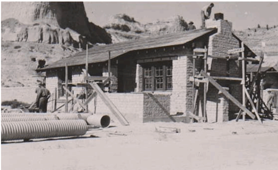
Ranger Residence under construction in 1939. Image courtesy of Scotts Bluff national Monument.
