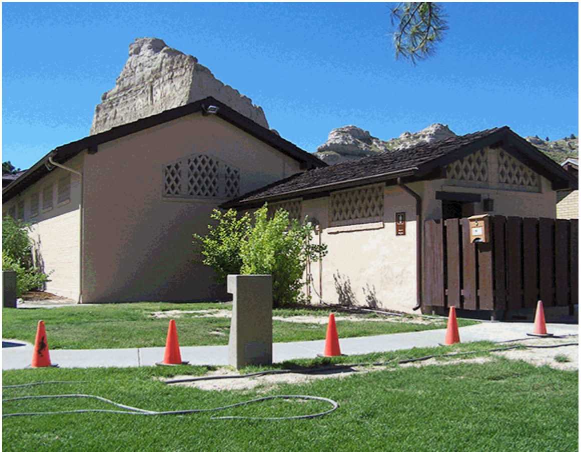
Comfort Station looking northwest (Reed 2014).
