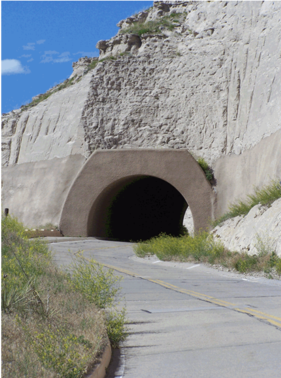
Summit Road Tunnel 3 looking north (Reed 2014).
