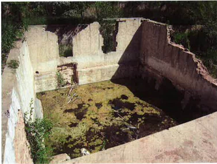
Figure 25. Minnekahta Spring, which emerges from pipes within an abandoned spa structure.
