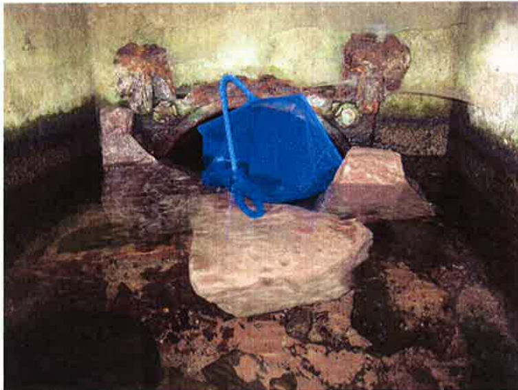
Figure 22. Interior of concrete structure at Evans Spring outlet, showing aquarium net over pipe outlet.
