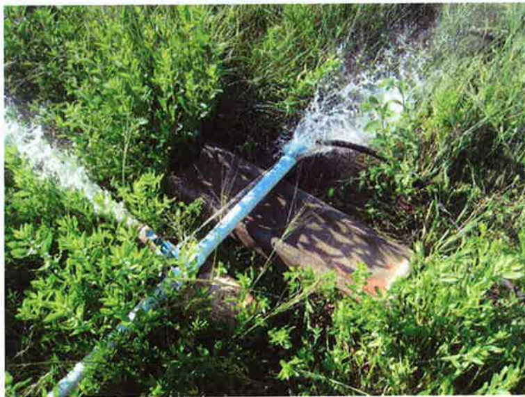
Figure 30. Park Well no. 2 outlet. A black hose is run up the pipe to shunt some of the flow to a 60 micron net.
