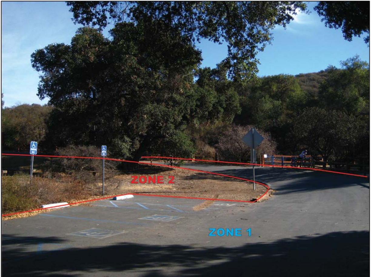
Figure A.5. Photograph of a parking lot with zone delineations that show the hardscape (Zone 1) and the maintained and unmaintained areas of Zone 2.
