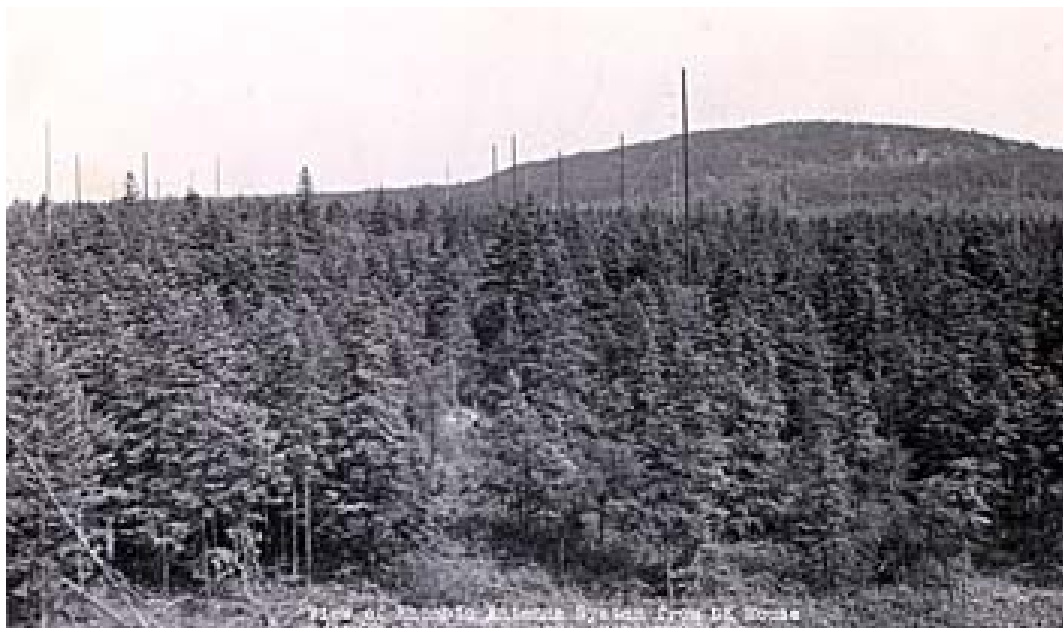
The caption to this photo, dated 9 Nov 1947, reads "View of Rhombic Antenna System from DK House" (Photo courtesy NSGA, Winter Harbor, 1947).
