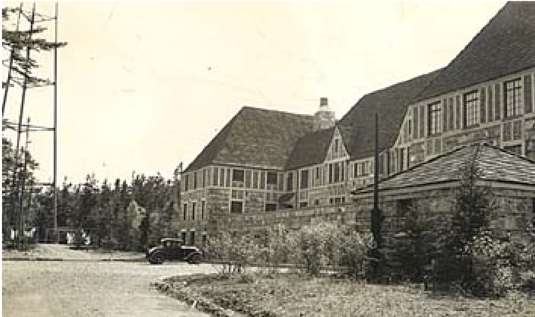
Grosvenor Atterbury-designed apartment building (Photo courtesy NSGA, Winter Harbor, ca. 1934).
