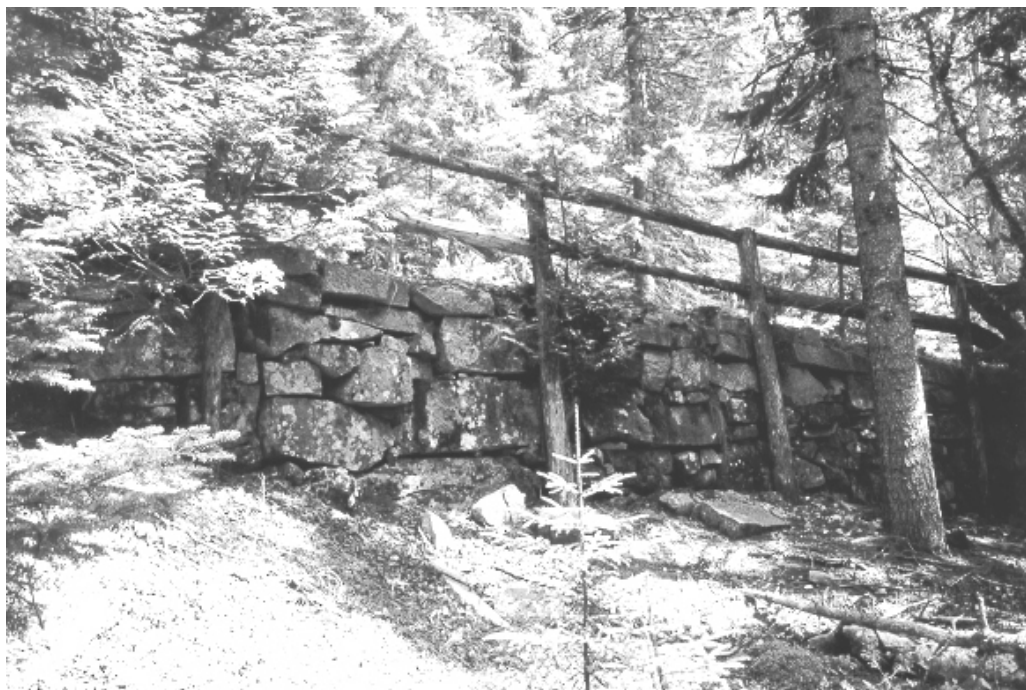
Rustic railing attached to retaining wall along Schoodic Head Road (OCLP, 2000).
