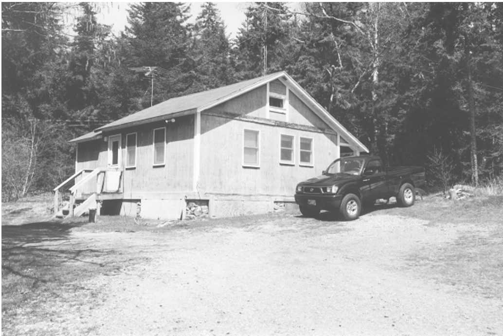
Schoodic Head ranger station (non-contributing) (OCLP, 2000).
