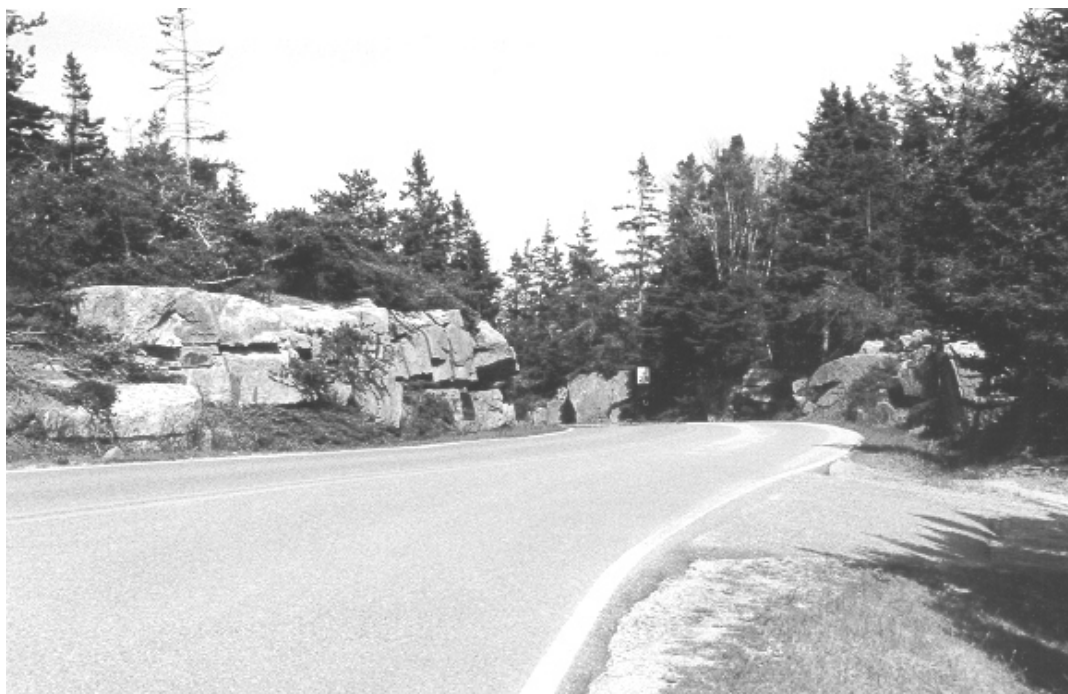
Ledge blasted to permit passage of loop road at grade level (OCLP, 2000).
