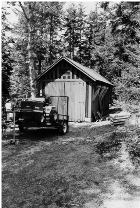
Schoodic Head ranger station garage (OCLP, 2000).
