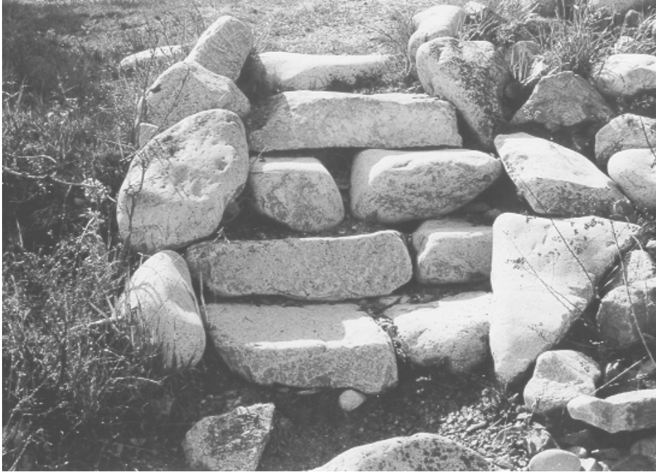
Steps fabricated of cobble between the loop road and a cobble beach (OCLP, 2000).
