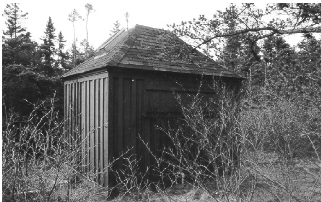
Schoodic Point pumphouse (OCLP, 2000).
