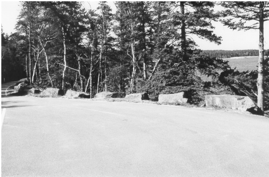
Coping stones lining a pulloff along the loop road (OCLP, 2000).
