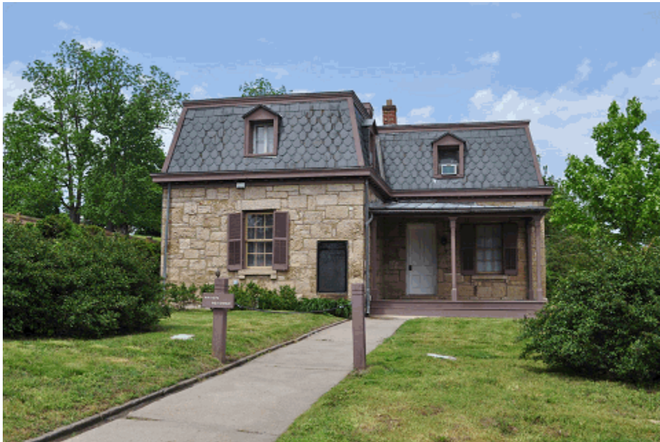
Figure 25. View looking north of the lodge, constructed in 1871, and the front concrete walk (OCLP, 2011).
