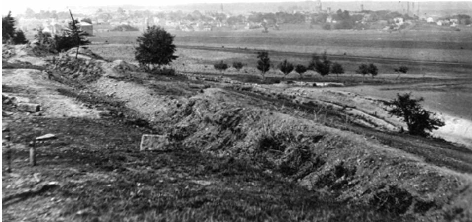
Figure 1. View looking northeast towards Fredericksburg from Marye's Heights on May 3, 1864. Note the stone wall at the foot of the hill and the trace of the Telegraph Road cut-off (Lafayette Blvd) entering the Sunken Road from the right (FRSP Archives).
