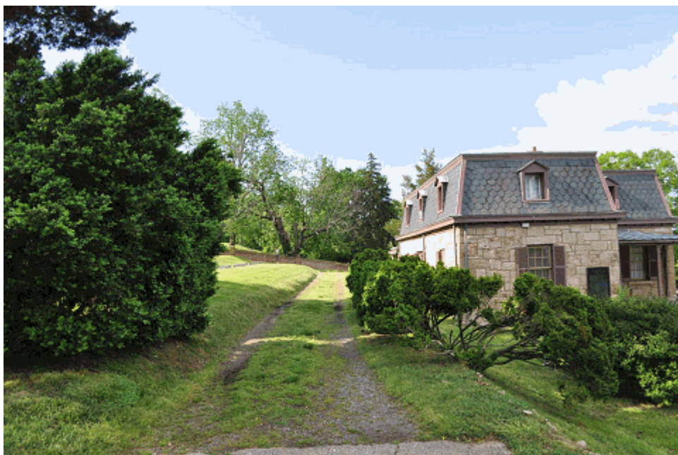
Figure 20. View looking north towards the service drive, boxwood hedge, and lodge (OCLP, 2011).
