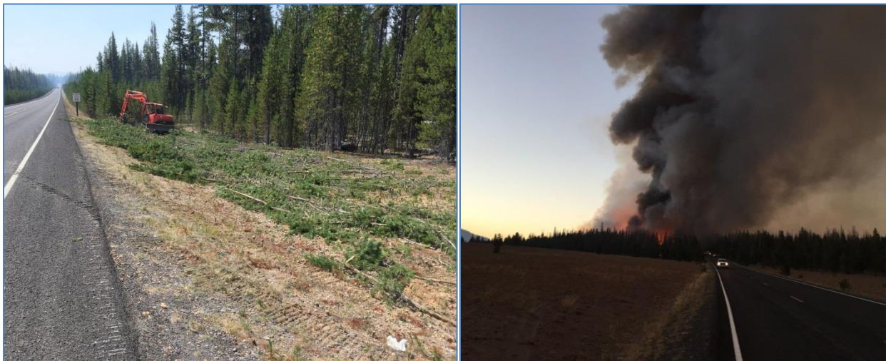
Figure 10. Left: Buzz-bar creating a fuelbreak along the North Entrance Road; Right: Burnout operations along the North Entrance Road north of the Pumice Desert. Photos by J. Beck.
